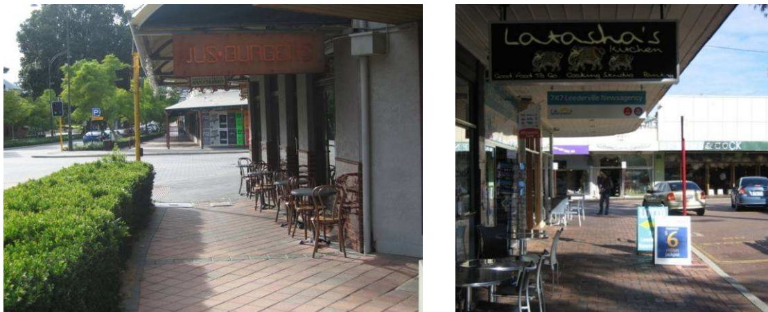
Figure 8 : Temporary obstructions on path
