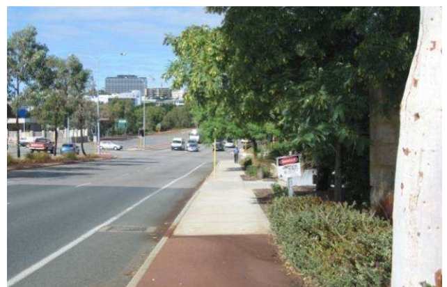
Pedestrian path adjacent to the kerb
