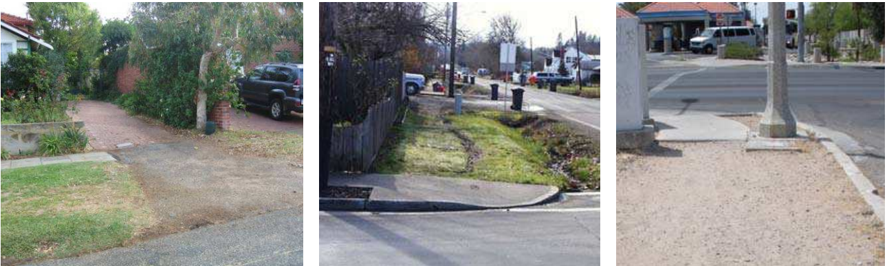
Figure 9: Abruptly ending footpath on missing (unpaved) section of footpath
