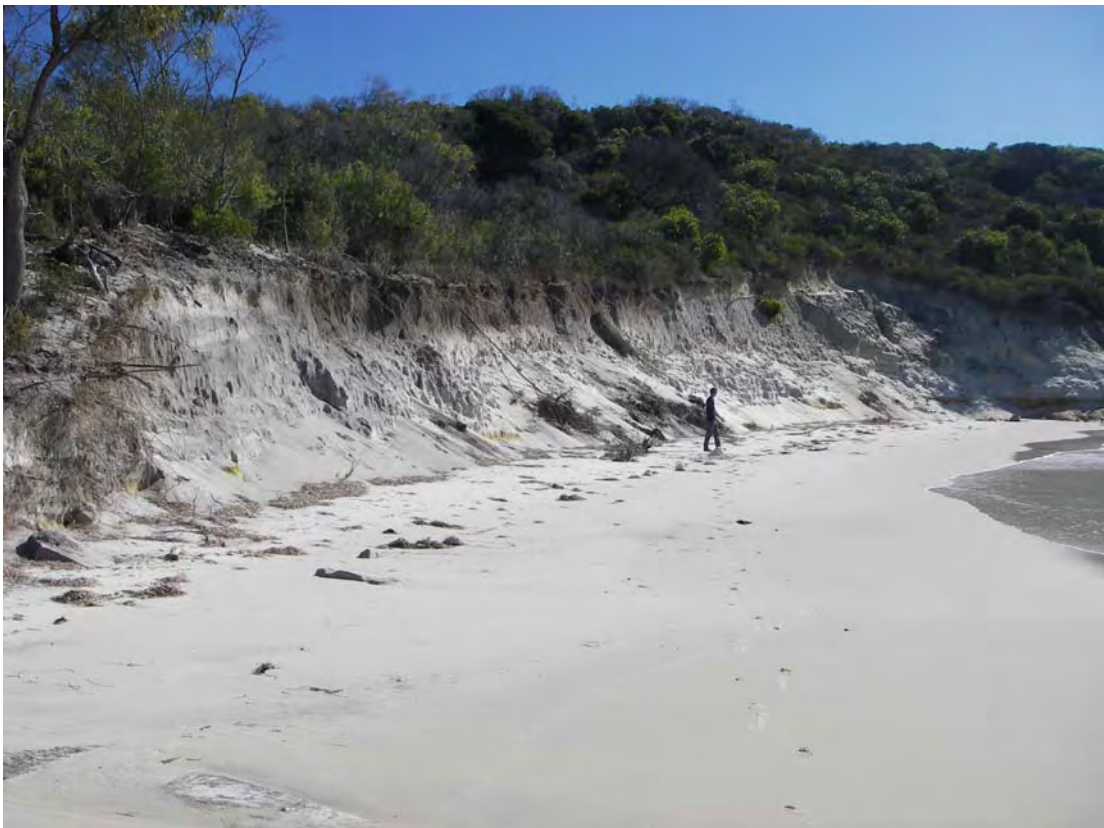
Figure 10: Photograph of the eroded scarp at the western end of Fishery Beach, 15 th March 2007.
