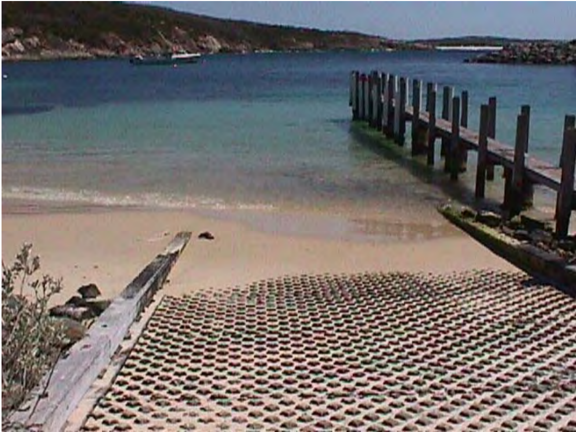
Figure 11: September 2006, boat ramps and finger jetty located at the eastern end of Fishery Beach. These ramps are prone to siltation which makes them difficult to use.
