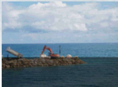
Construction of the Breakwater
