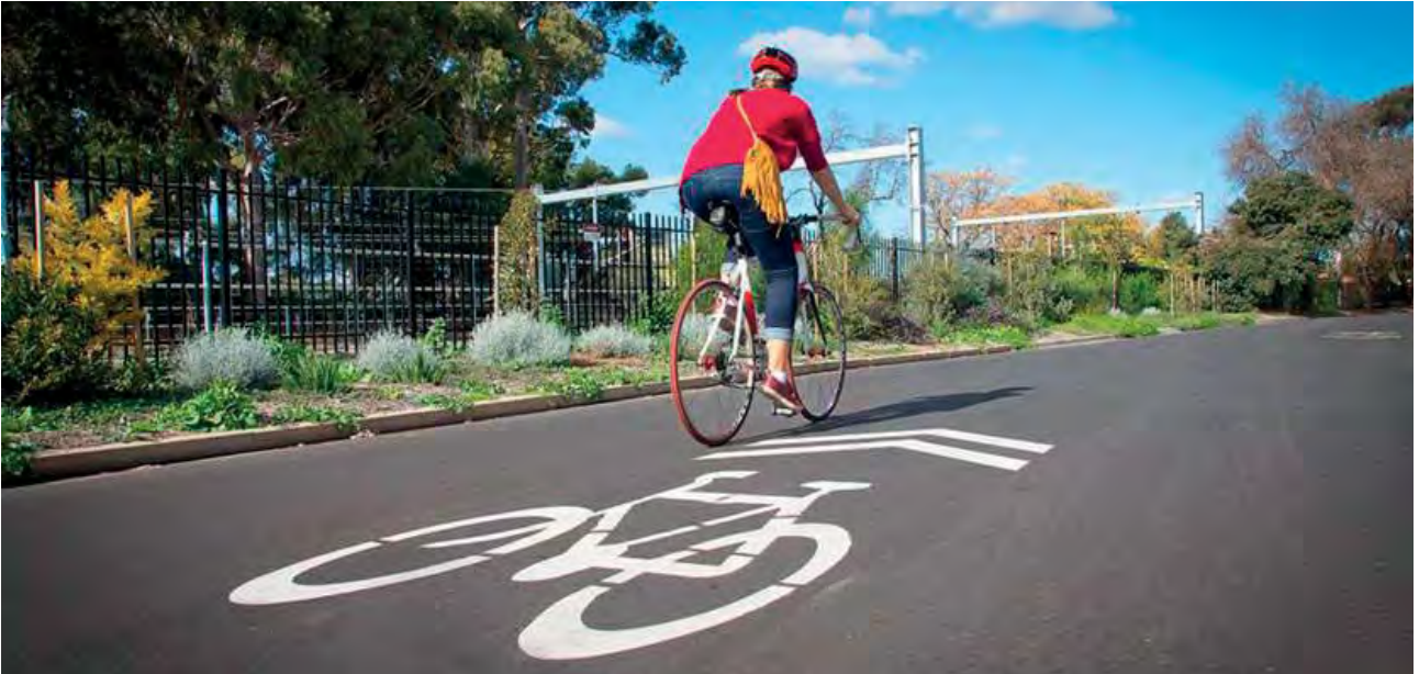
Figure 10: A sharrow (road marking) in Adelaide.
