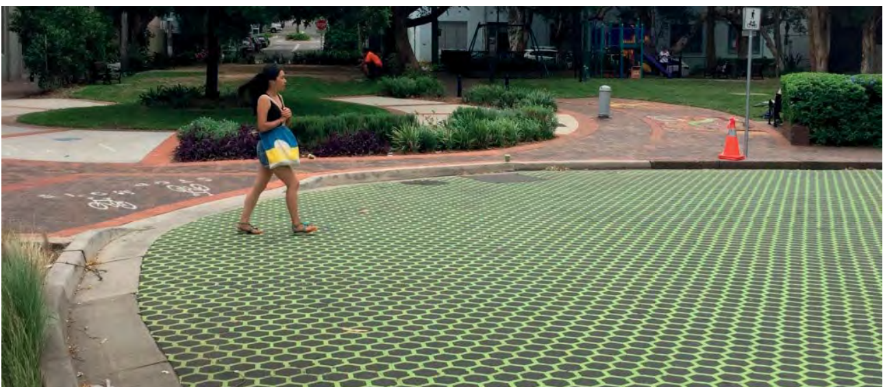
Figure 18: Use of honeycomb road markings without cyclist priority; shared path sections
