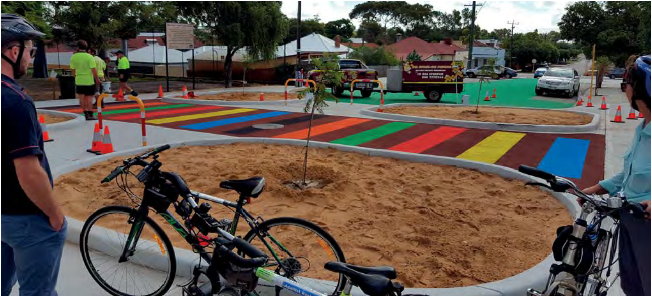
Figure 8: Inspecting the freshly painted crossing of the bike boulevard in Bayswater linking the primary school to its oval
