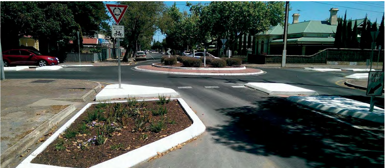
Figure 11: Changes to roundabout approaches
