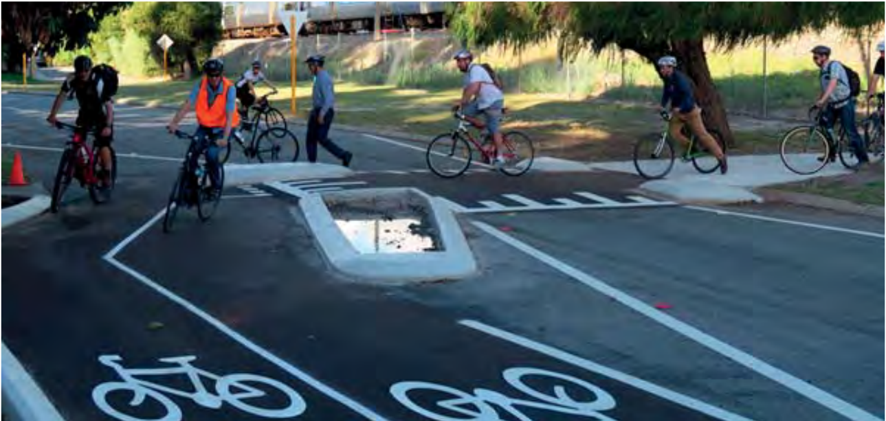
Figure 6: Crossing a single-lane slow point on Railway Parade, Bayswater
