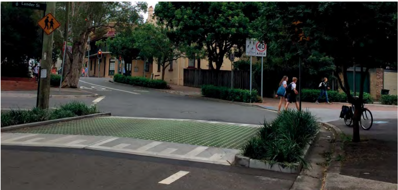
Figure 17: Flat top speed humps, planters, bike symbol road markings and 40km/h limits
