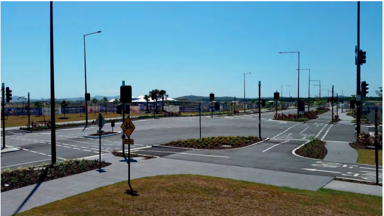
Figure 19: Dutch-style protected intersection in Caloundra, Queensland
