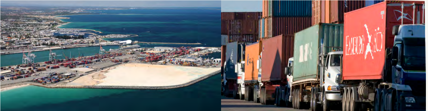
Land newly reclaimed at Rous Head as part of the Inner Harbour deepening will be used for port-related purposes.
