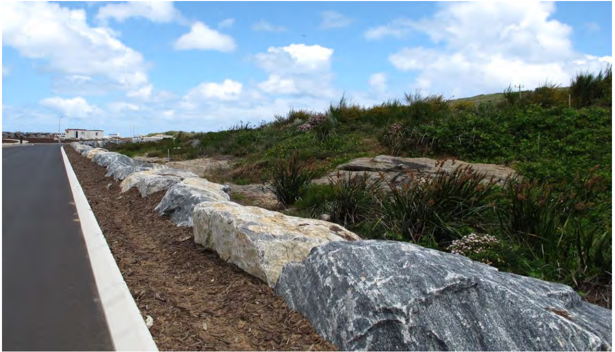
PLATE 11 Rock wall along Rehabilitaiton Block - preventing access
