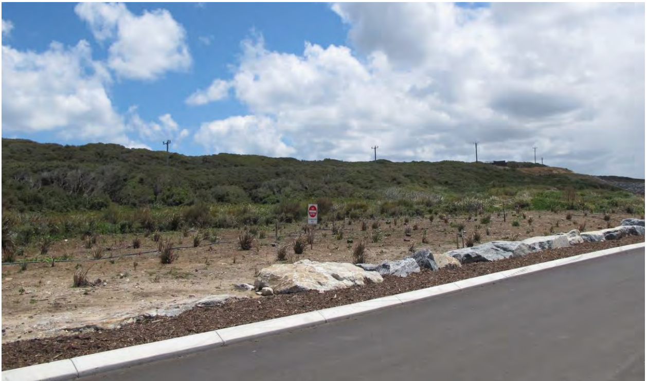
PLATE 2 2014 Rehabilitation Block - Old Site Office
