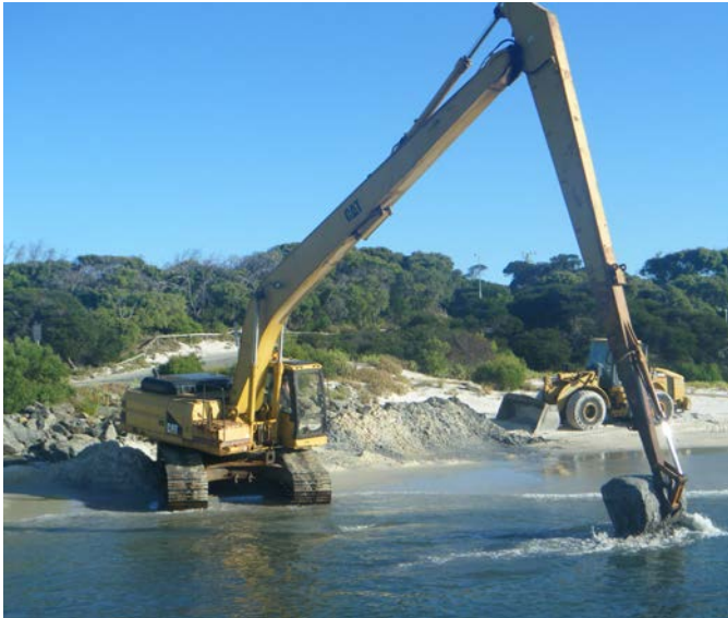
Excavation from shore – Bremer Bay 2010
