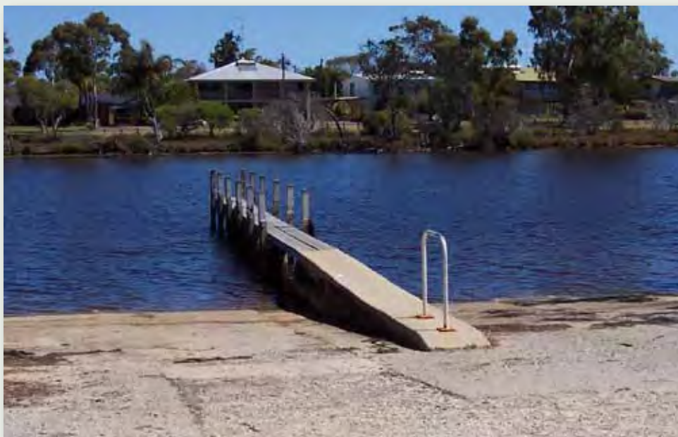
Figure 11. Typical two-lane boat ramp with finger jetty on the Serpentine River
