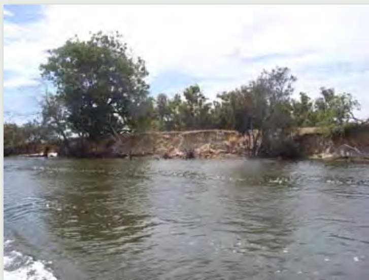
Figure 9. Example of riverbank erosion
