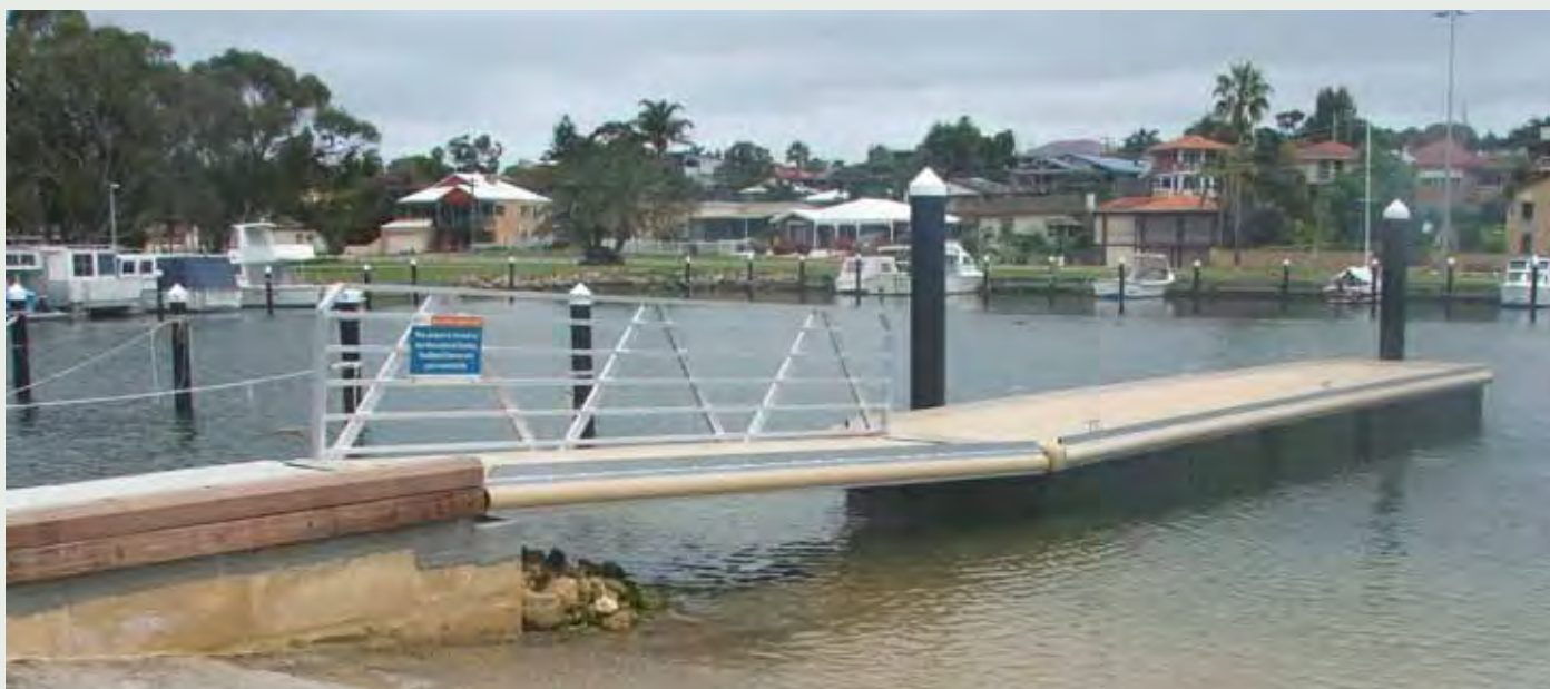
Figure 19. Universal access floating pontoon at Mary Street Lagoon boat ramp
