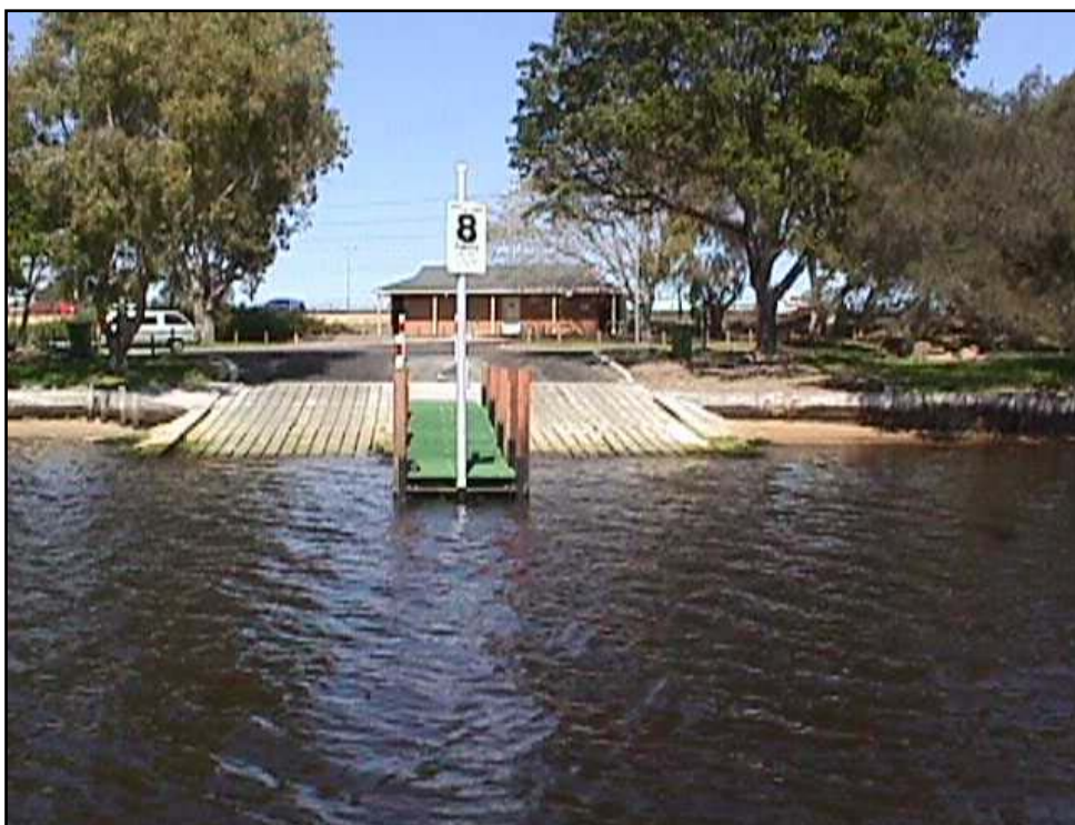
Figure 2: Typical Two-Lane Ramp With Finger Jetty On The Swan River
