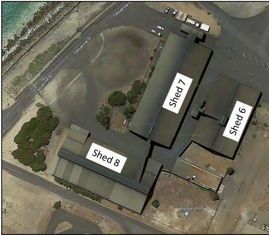
Photograph 1 Outer Harbour Port Shed 6, 7 & 8
