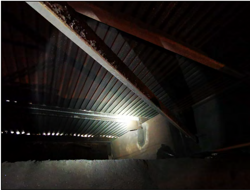
Photograph 88 Wall Girt Missing
