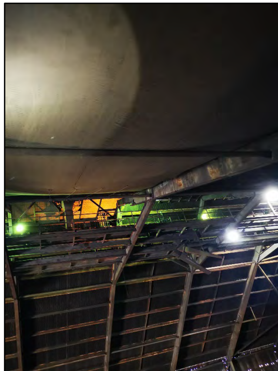
Photograph 32 Bay 6 in Shed 6 was Covered with Tarpaulin
