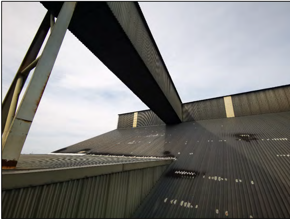
Photograph 132 Roof Sheeting and Conveyor System
