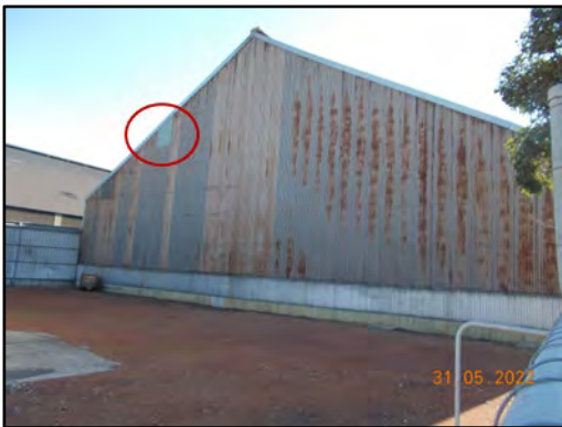
Photograph 42 Shed 6 South Side on 31 May 2022
