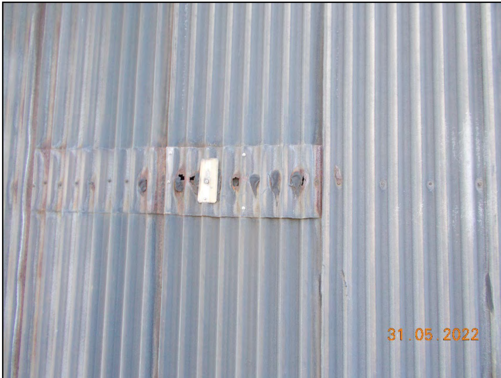
Photograph 50 Patching to Wall Sheeting
