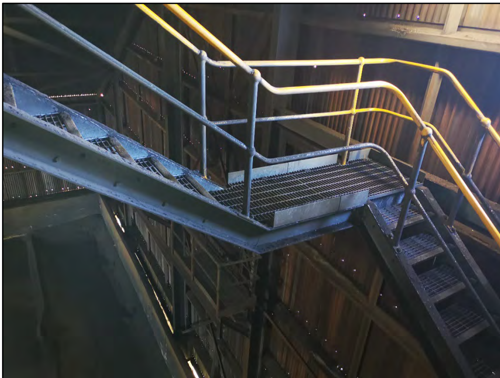
Photograph 30 Stairway Inside Shed 6
