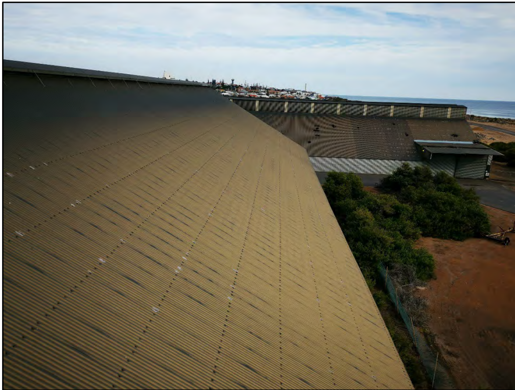
Photograph 56 No Significant Corrosion
