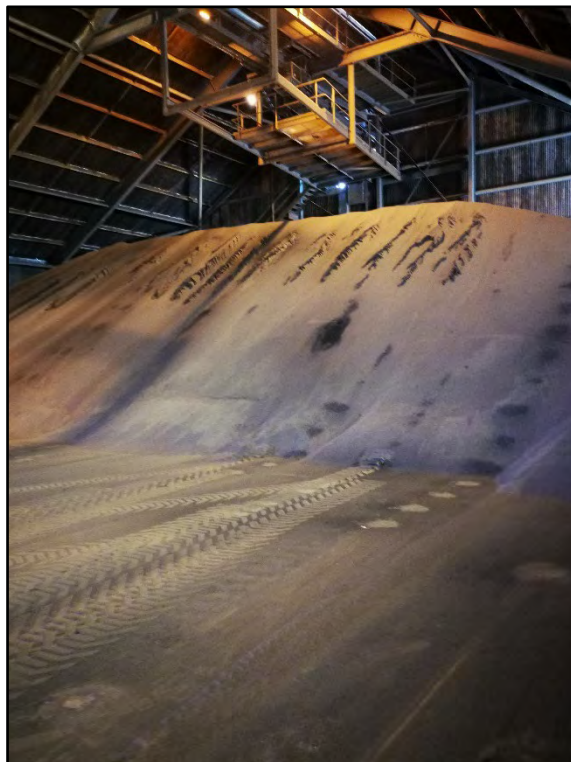
Photograph 119 No Slab Damage or Crack Observed
