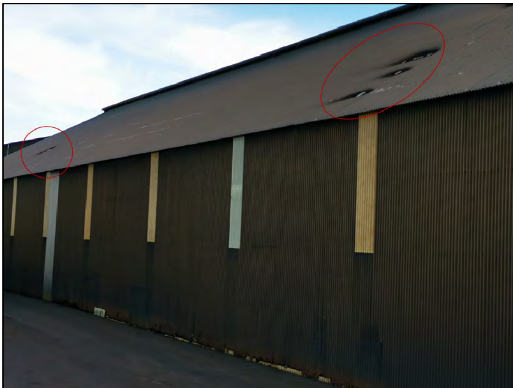
Photograph 57 Patch Work on Roof Sheeting
