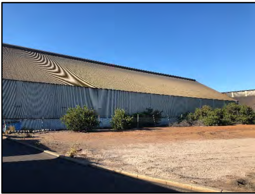
Photograph 59 Shed 7 Eastern Side on 31 May 2022
