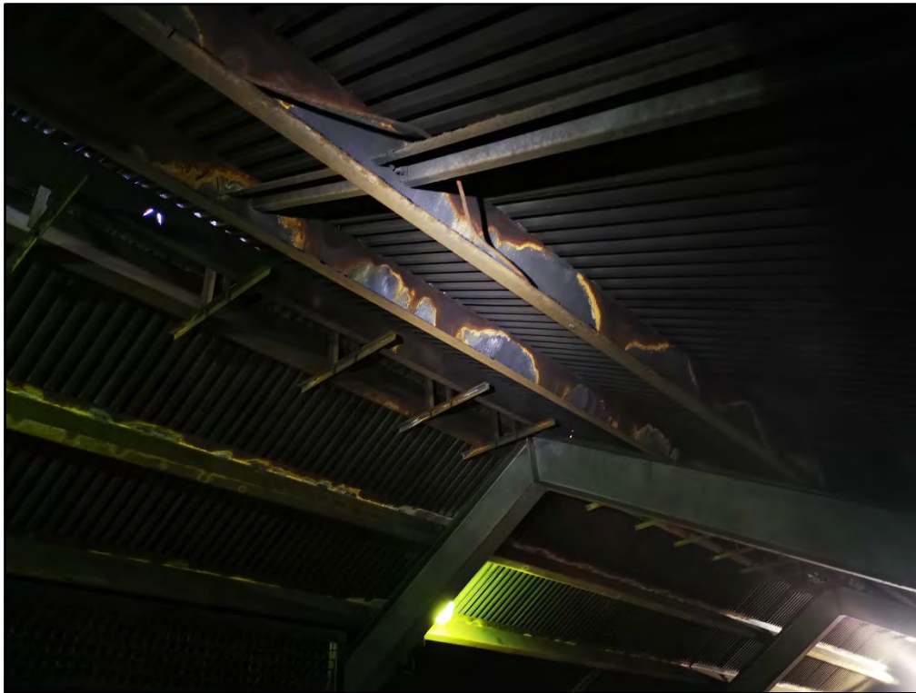
Photograph 27 Surface Corrosion of Purlins
