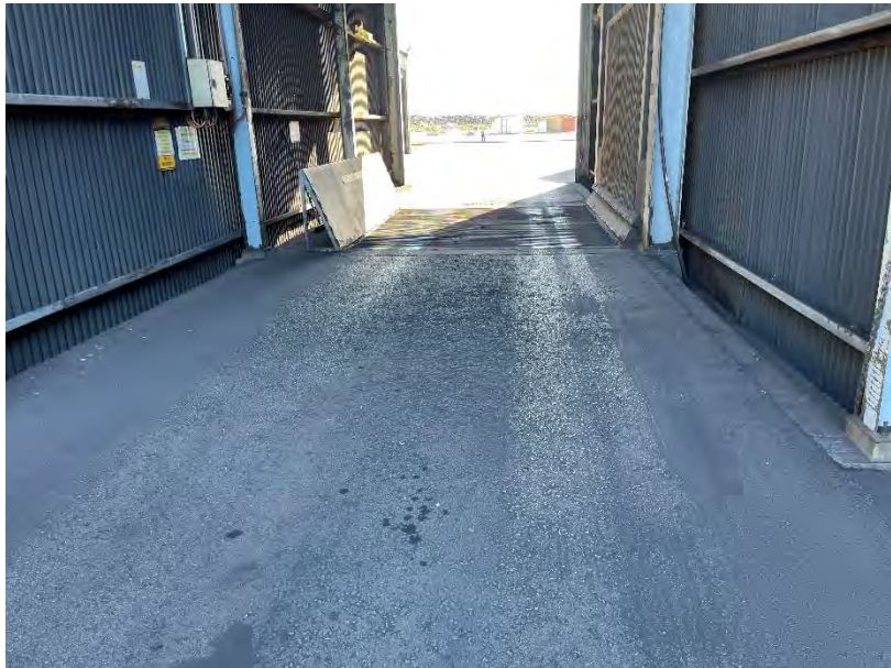
Photo 40: View to Road Hopper, roller shutter on north side only
