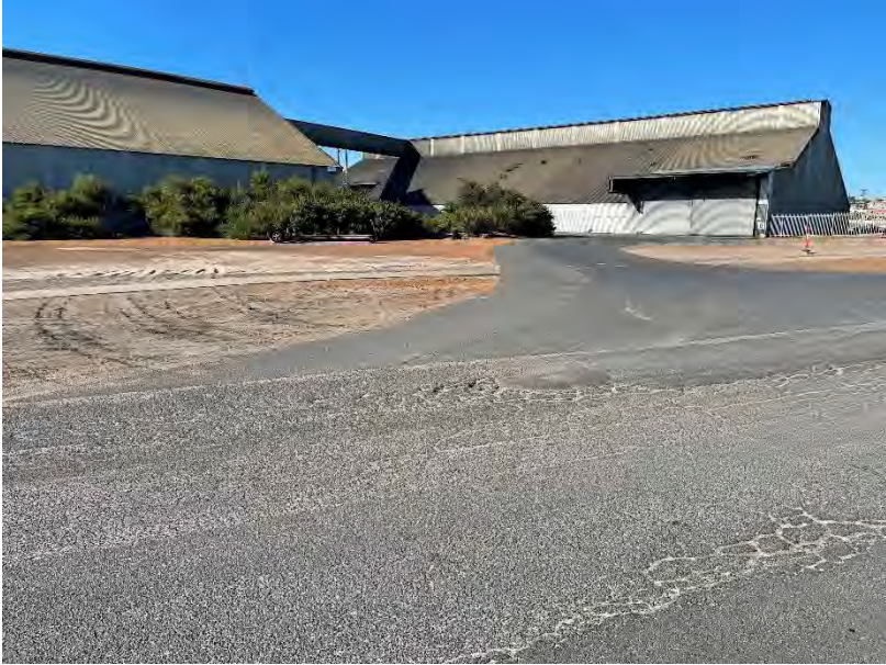
Photo 01: View to Shed 8 (right) Shed 7 (left)
