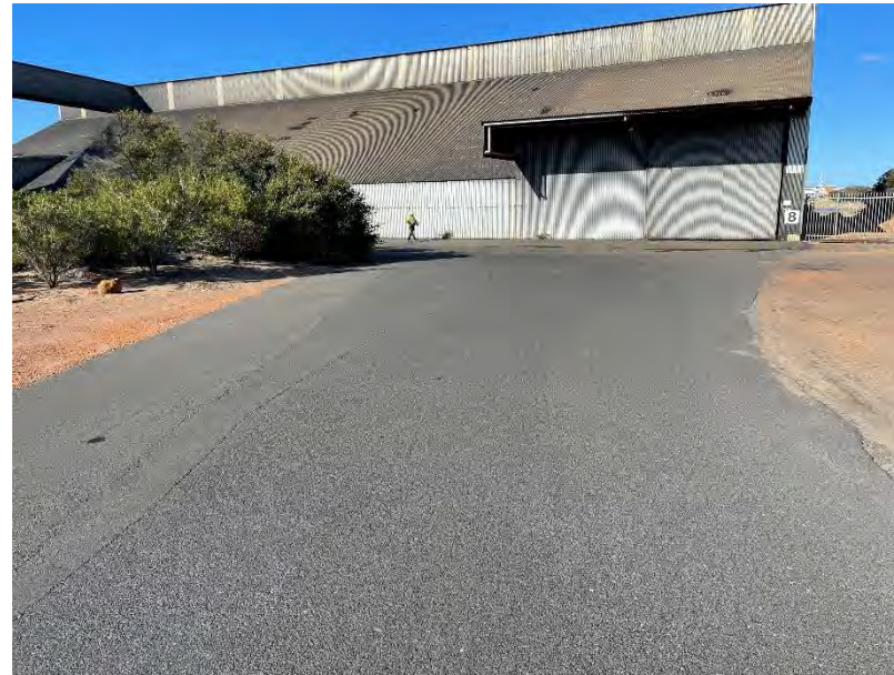
Photo 19: Road surface to Shed 8 in good condition
