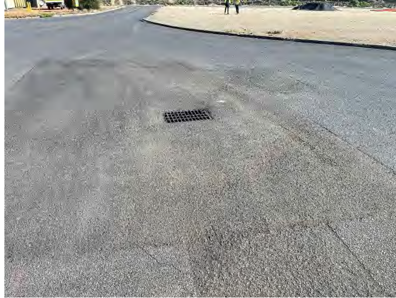
Photo 59: Surface grated inlet pit lid in good condition
