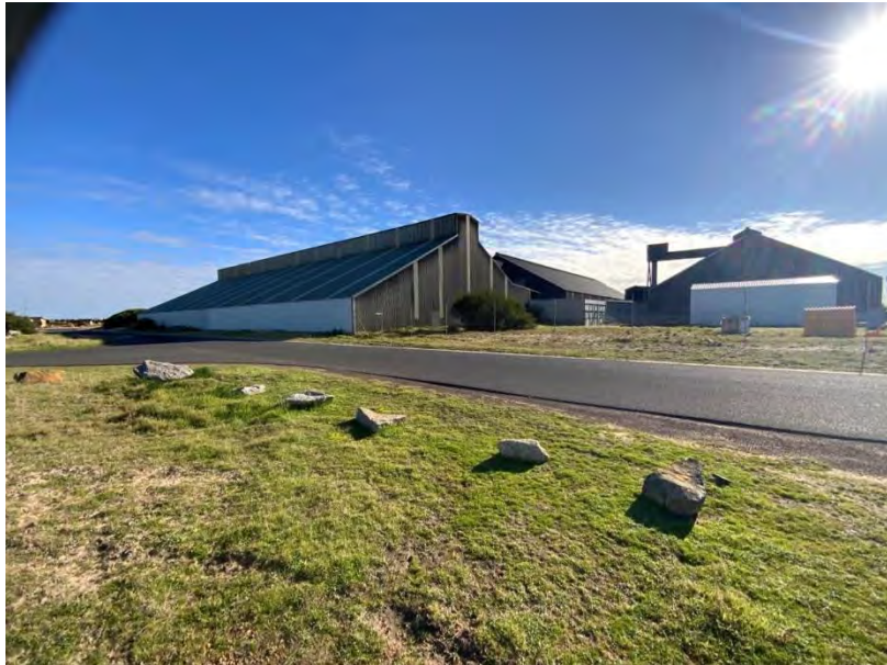
Photo 112: From outside to Shed 8 (left) and Shed 6 (right)
