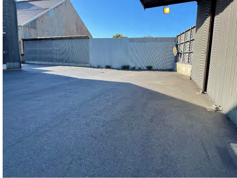
Photo 33: View to Shed 8 (right) Shed 7 (left) Shed 6 (middle)
