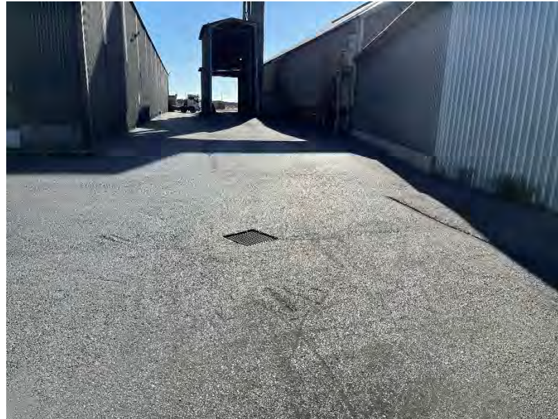
Photo 35: Surface grated inlet pit lid in good condition
