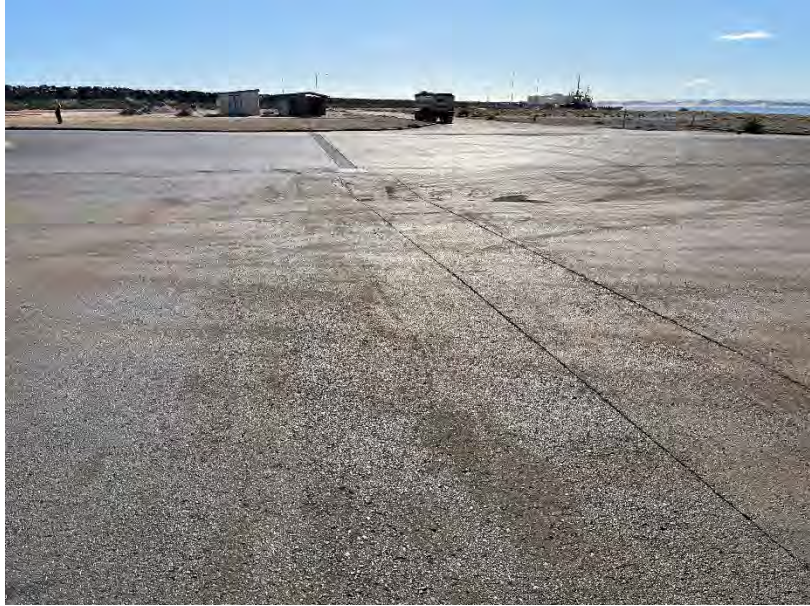
Photo 50: Generally drains well (By site supervisor)
