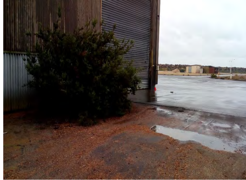
Photo 103: View to Shed 6, well draining soil with some small puddles
