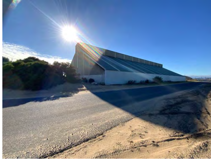
Photo 111: From outside to Shed 8
