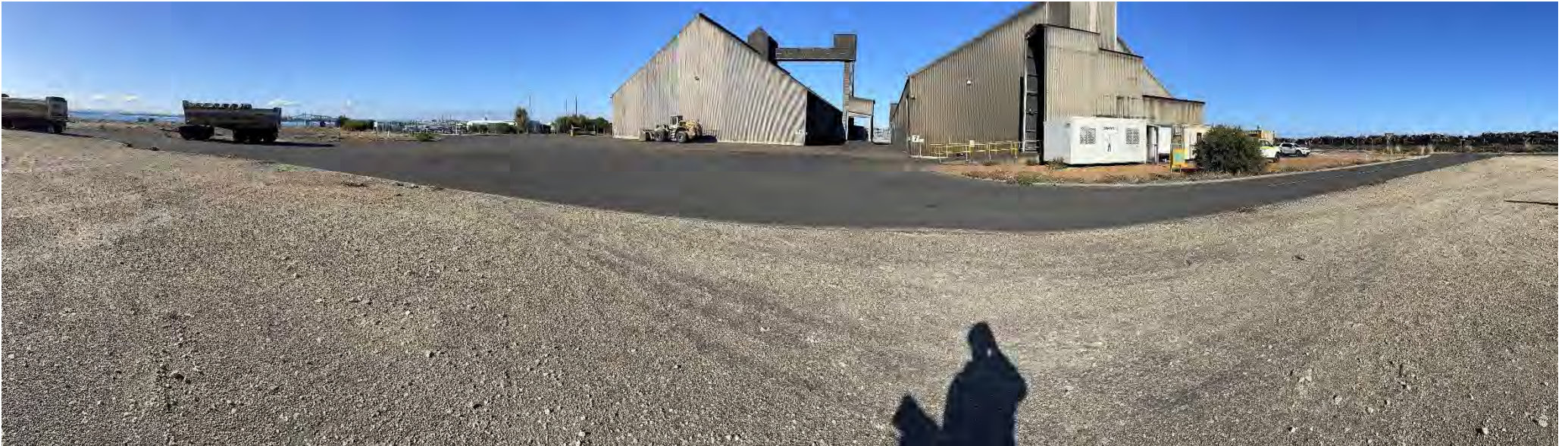
Photo 63: View of Shed 7 and site shed (right) Shed 6 (left)
