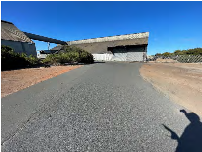
Photo 18: Road surface to Shed 8 in good condition
