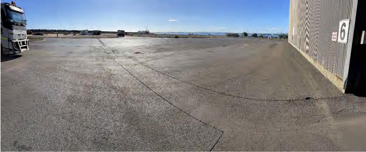
Photo 47: Road surface in good condition with some minor repair required.
