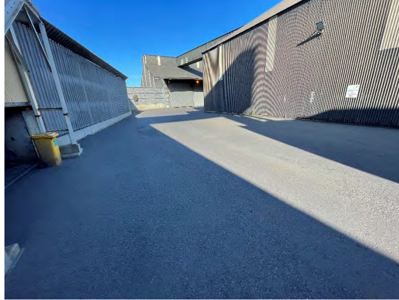
Photo 37: View to Shed 8 (middle), Shed 7 (right) Shed 6 (left)
