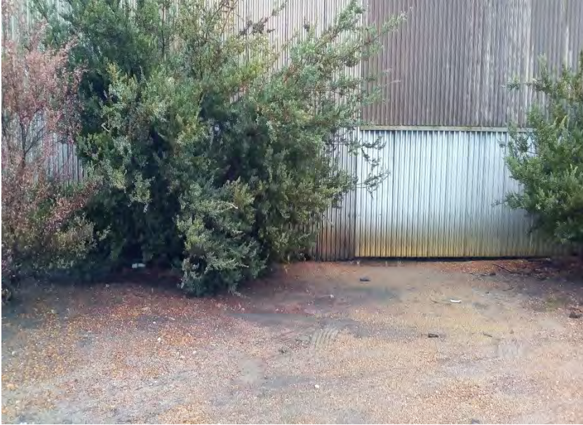
Photo 102: View to back of Shed 6, well draining soil (wet condition)
