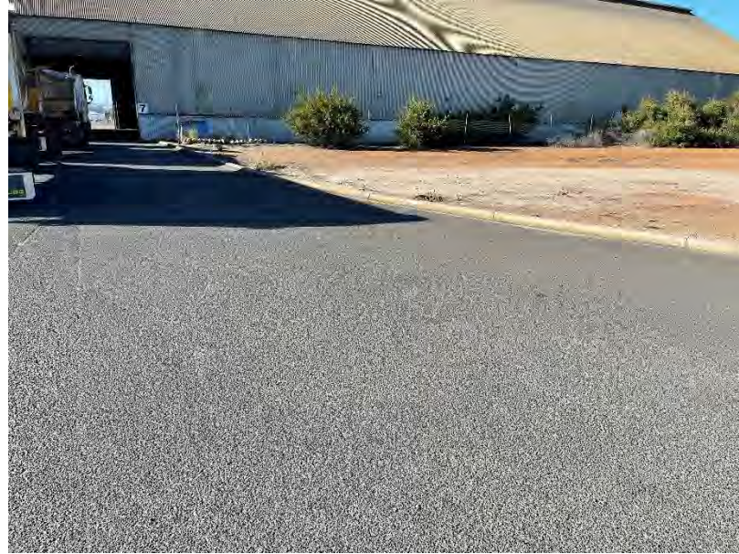
Photo 92: Road surface is generally in good condition
