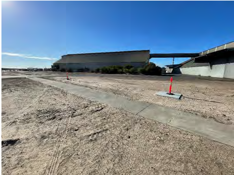
Photo 15: View to Shed 8 (right) and Shed 7 (left)
