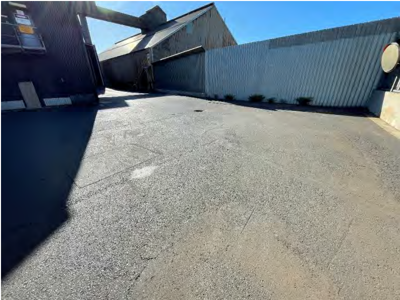
Photo 34: View to Shed 7 (left) Shed 6 (right)
