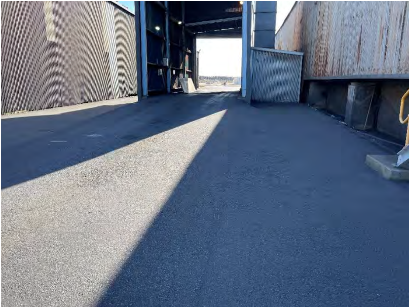
Photo 38: View of road hopper and Shed 7 (left) Shed 6 (right)
