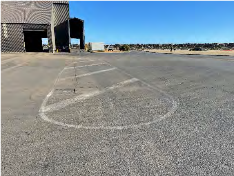
Photo 56: Reinstatement of linemarking (if required for new proposal)
