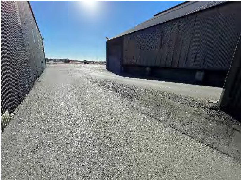
Photo 42: View to Shed 7 (left) Shed 6 (right), steep slope at Shed 6
