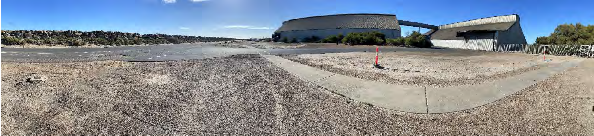
Photo 17: Shed 8 (right) Shed 7 (left)
