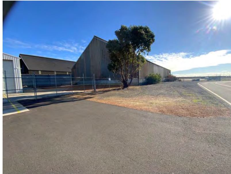
Photo 113: From outside to Shed 7 (left) and Shed 6 (right)
