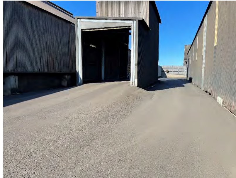
Photo 43: View to Shed 7 (right) Shed 6 (left), steep slope at Shed 6
