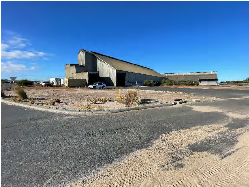
Photo 80: Damaged kerb due to heavy vehicle sweeping through kerb
