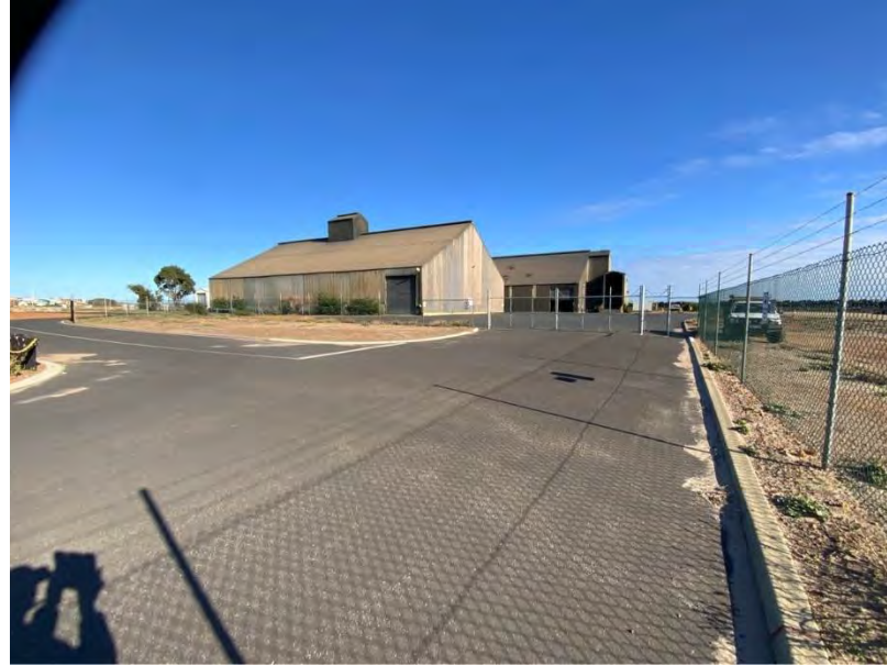
Photo 115: From outside to Shed 6 (left) and Shed 7 Right)
