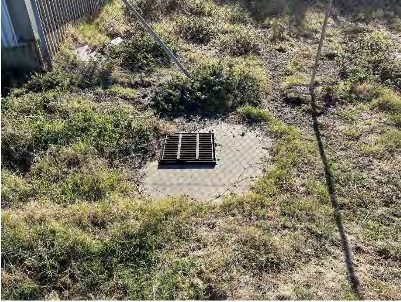
Photo 64: Surface water grated inlet pit lid outside Shed 6
