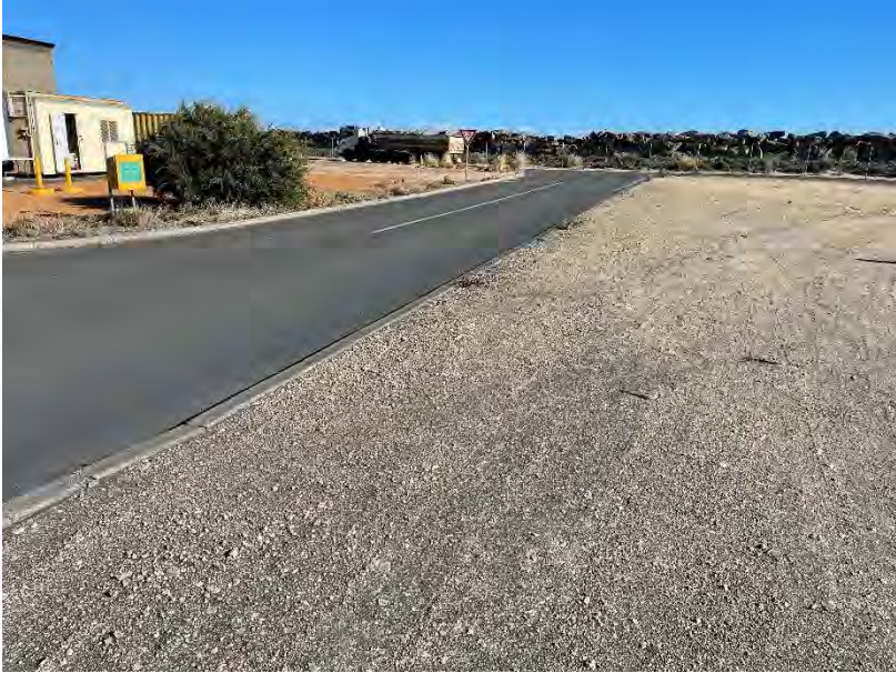
Photo 62: Road surface is in good condition.
