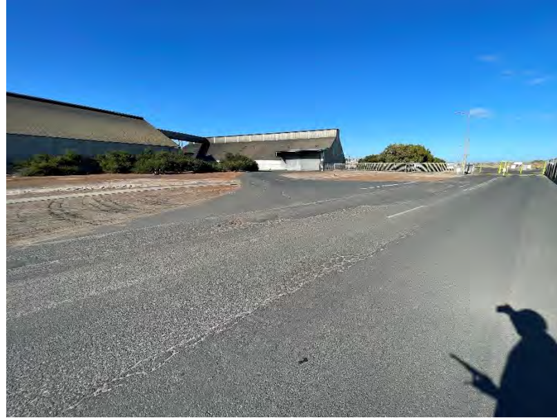
Photo 99: Access road to Shed 8 is in good condition.
