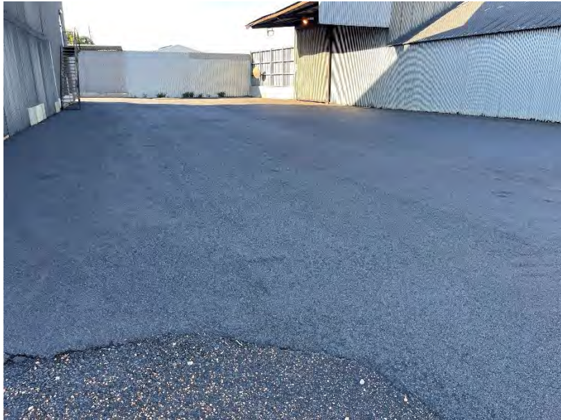
Photo 30: Road surface in good condition
