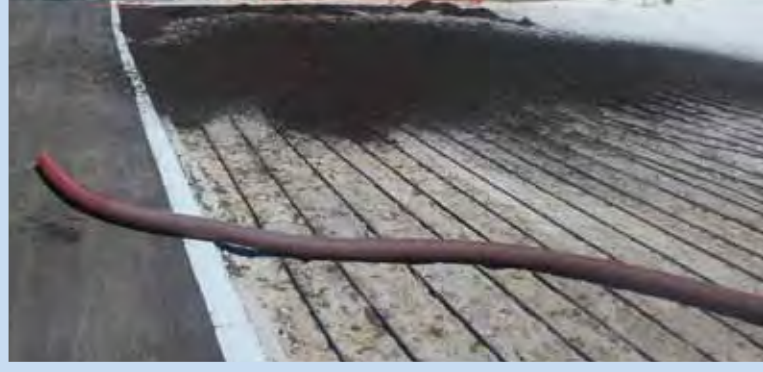
Final stages of landscaping construction works
