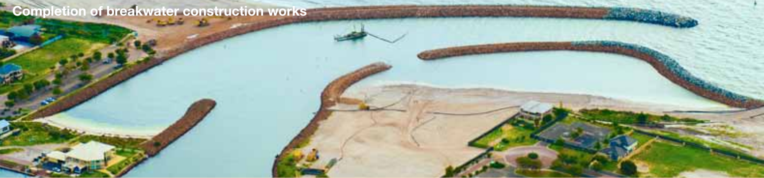
Completion of breakwater construction works
