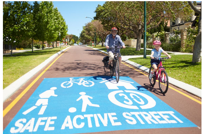
Blue patch mid-block, with narrowed carriageway
