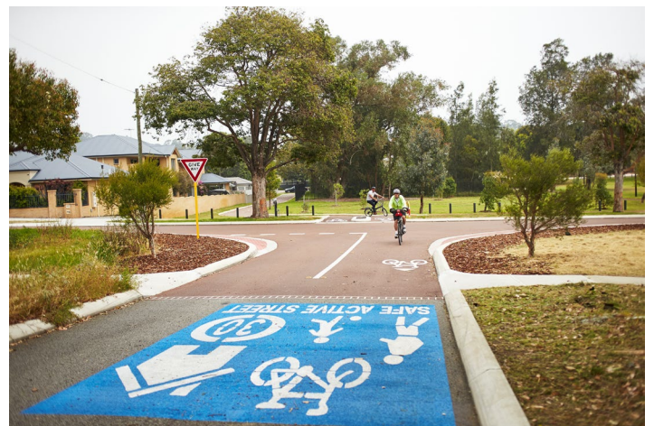
Shared path connection, blue patch after intersection and riders in primary position
