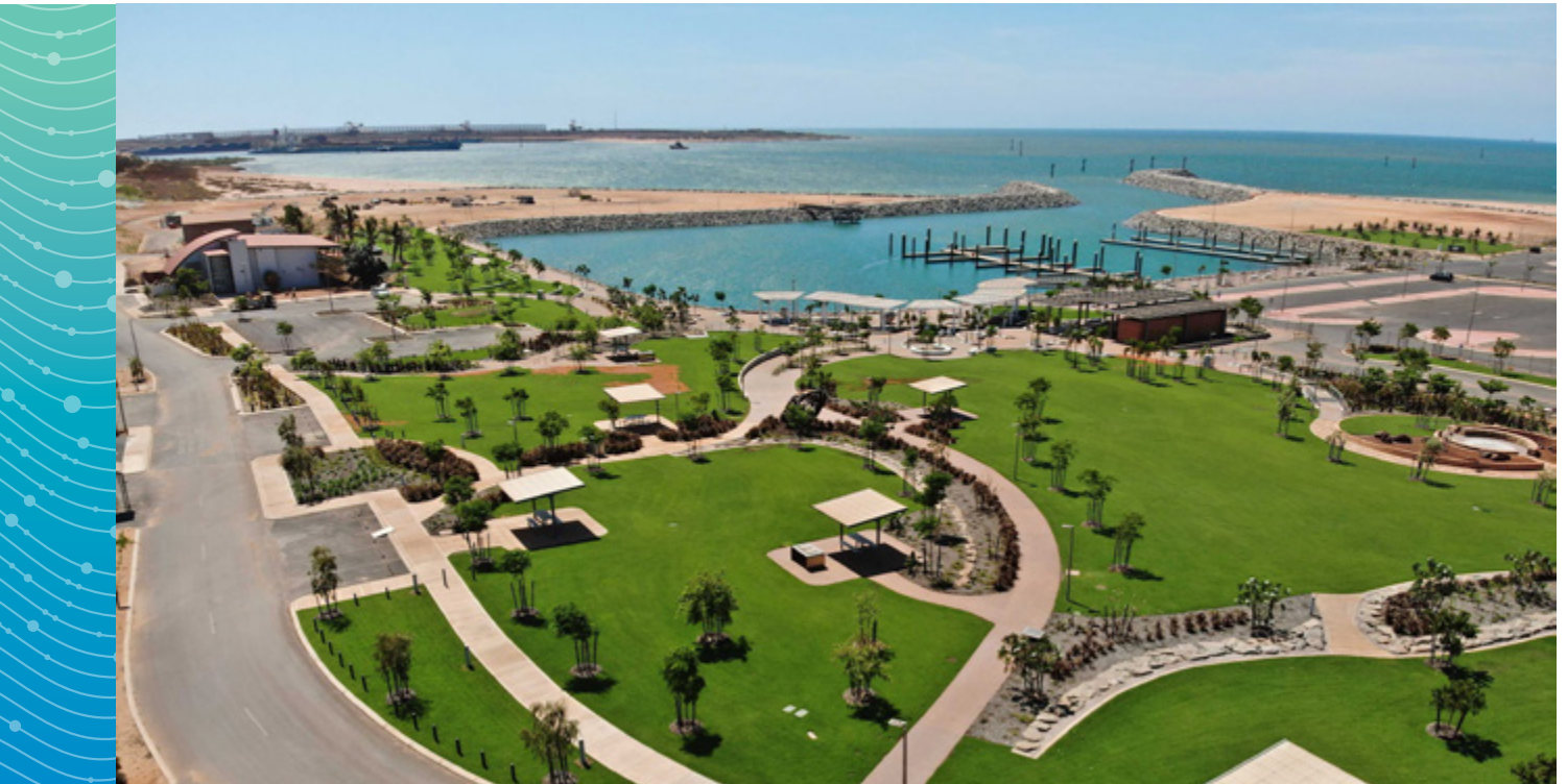
Cover photograph: New boat pens at Geraldton (Batavia Coast) Marina Above photograph: Spoilbank Marina, Port Hedland
