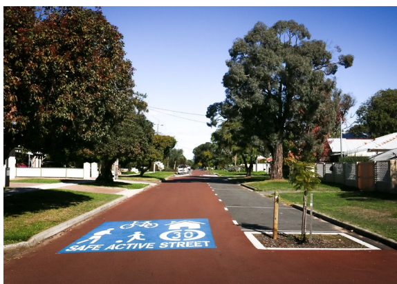
Combinations of treatments: formalised parking, tree plantings, blue patch
