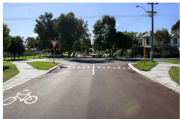
Filtered permeability and wayfinding at transition to road closure
