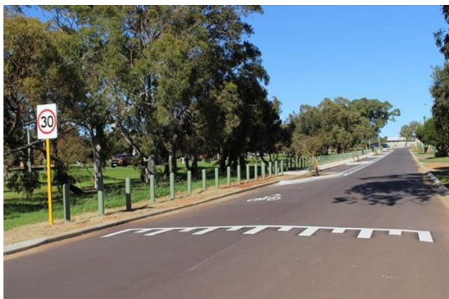
Raised intersection plateau and 30 km/h signage
