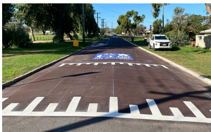
Road hump and blue patch at entry point
