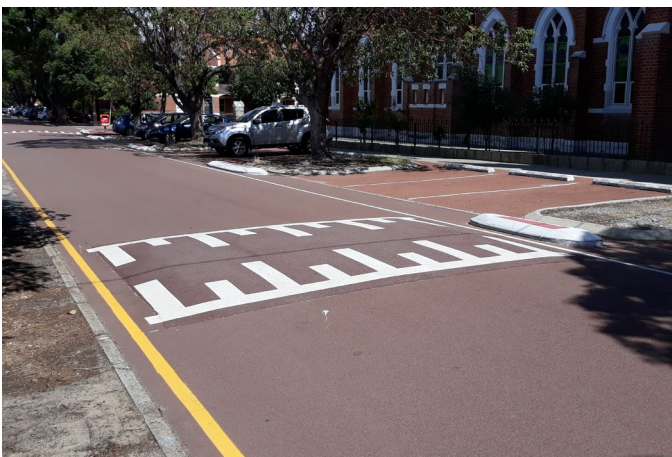
Road hump and kerb build outs
