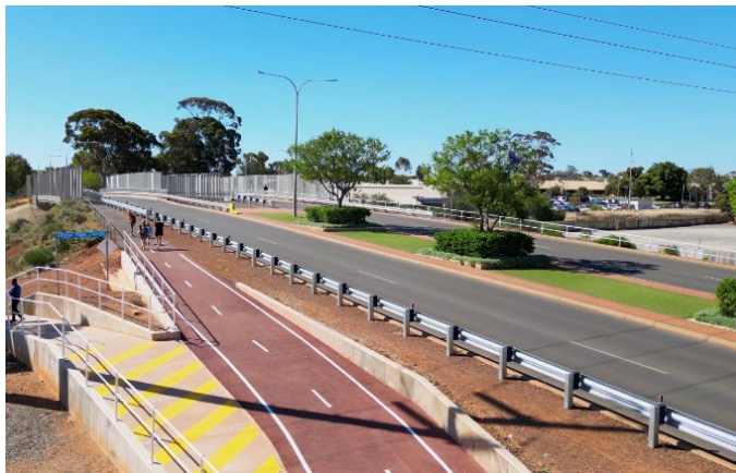
Keenan Street and Maritana Street Shared Path (Stage 1). Photo credit: City of Kalgoorlie-Boulder
