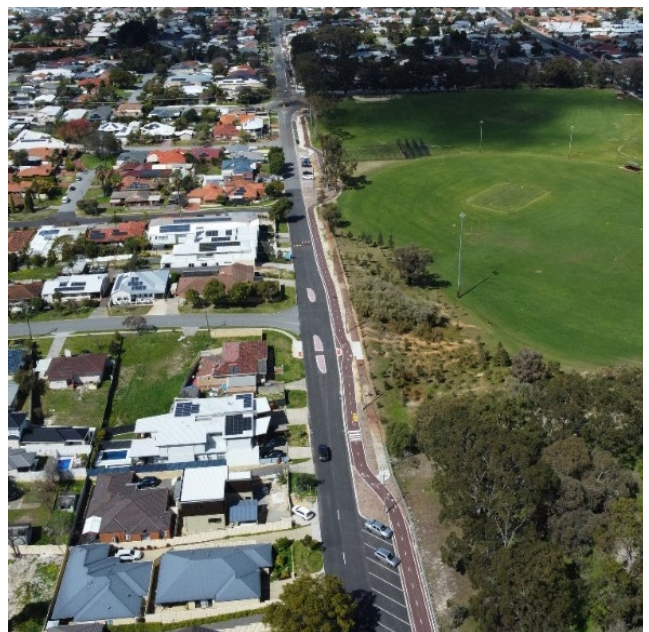
Drake Street Separated Bike Path. Photo credit: City of Bayswater
