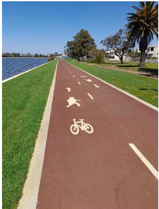
Frank Buswell Foreshore Shared Path Upgrade. Photo credit: City of Bunbury
