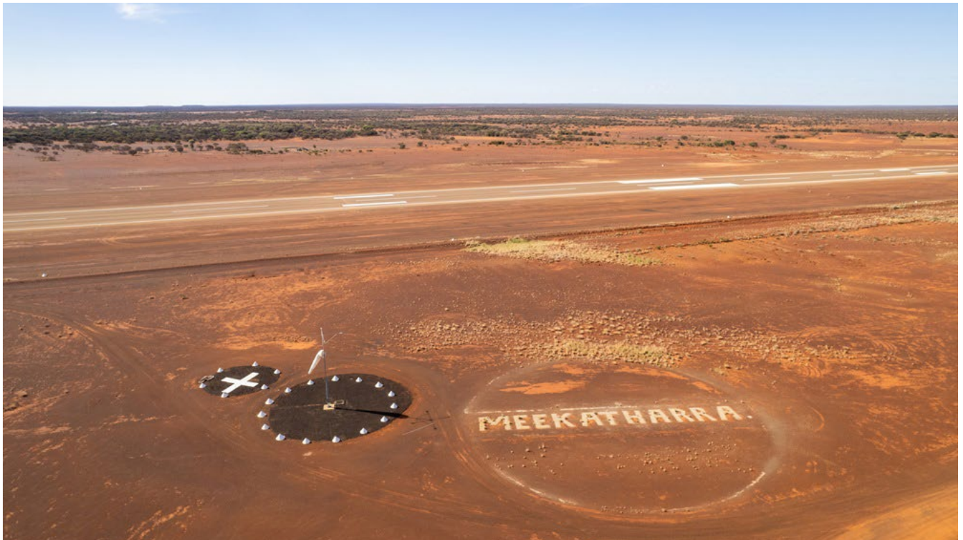
Completed runway sealing works at Meekatharra Airport, 2024
