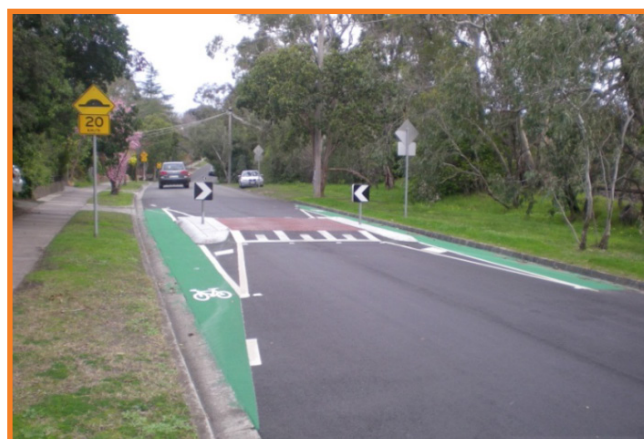
One-way slow point with bicycle-bypass facilities 3
