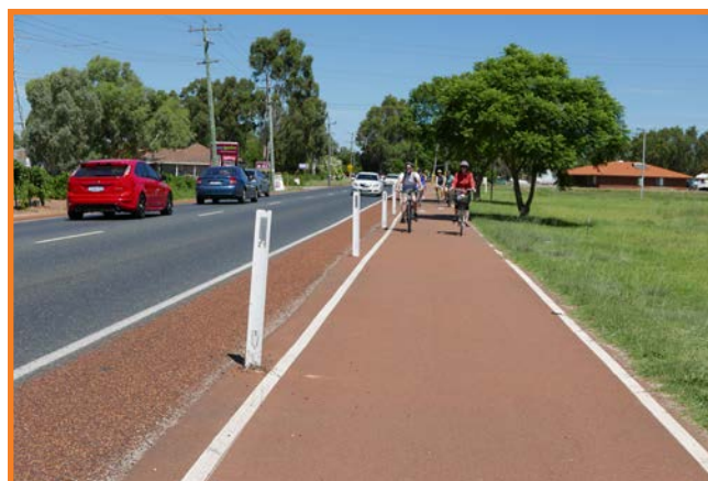
Bi-directional bike lane separated with bollards
