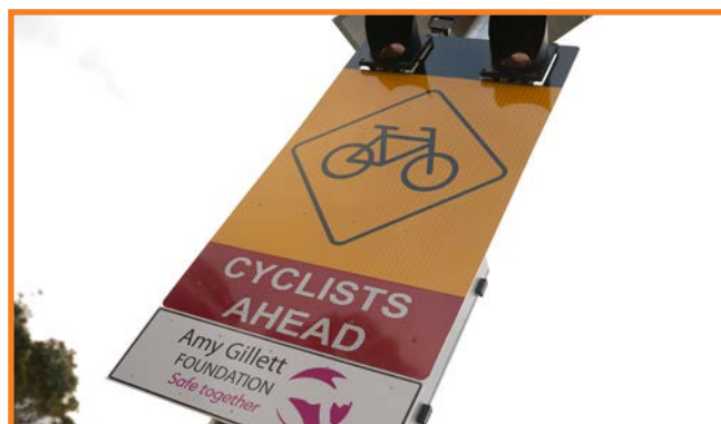
Dynamic flashing warning lights (Victoria)
