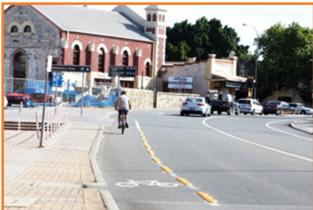
Bike lane separated with mountable plastic kerbing
