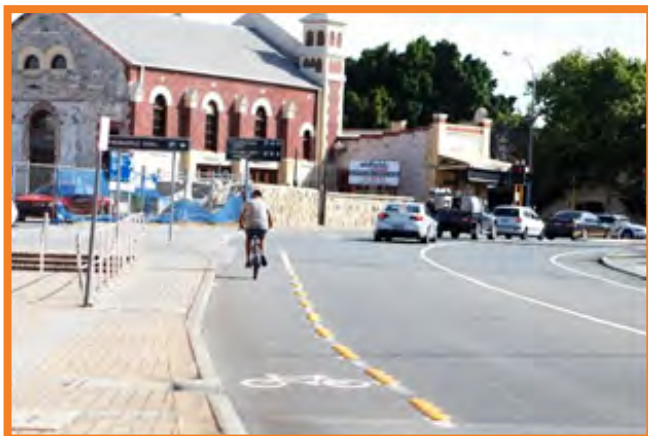
Bike lane separated with mountable plastic kerbing
