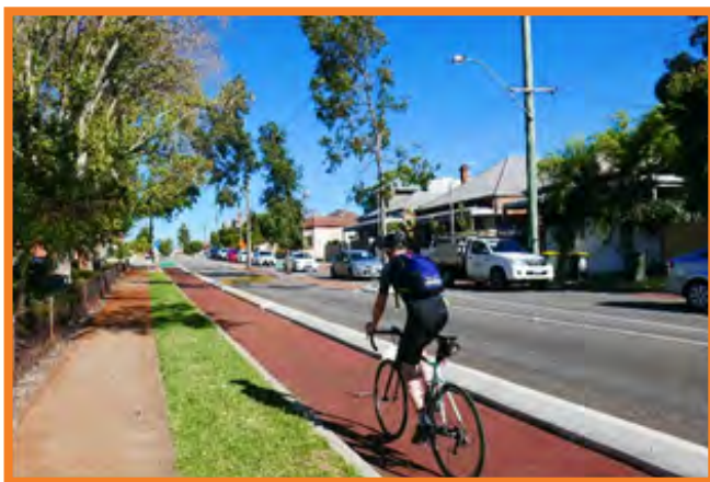
Bike lane protected with concrete kerb
