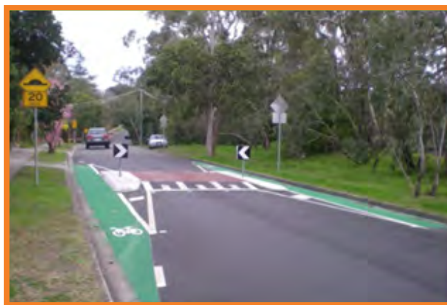
One-way slow point with bicycle-bypass facilities
