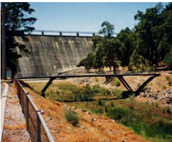
Dam wall that forms Mundaring Weir
