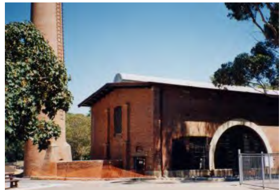
No. 1 Pump Station at Mundaring Weir
