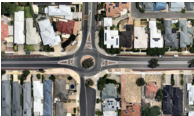
Figure 38: Roundabout with single leg full closure.
