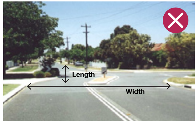
Figure 45: Modified T-intersection with normal priority. (Source: MRWA).
