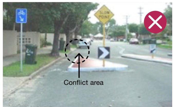
Figure 23: Angled two lane slow point with cycle bypass abruptly terminating.
