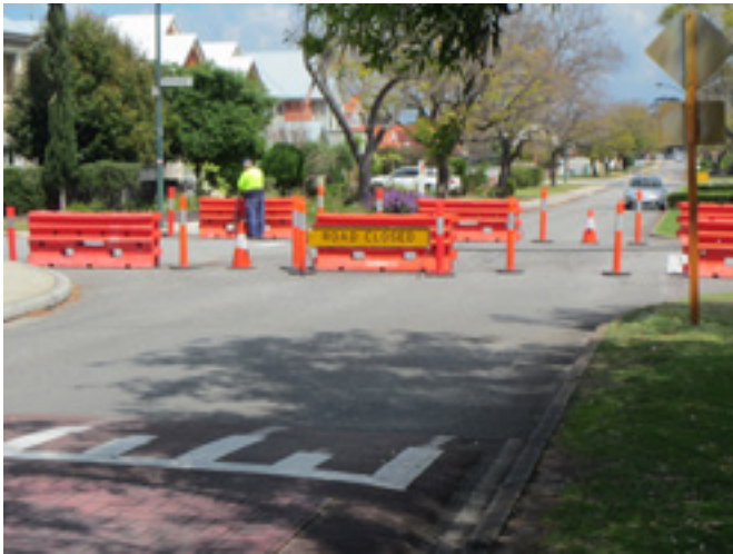
Figure 34: Macrae Road before road closure treatment.
