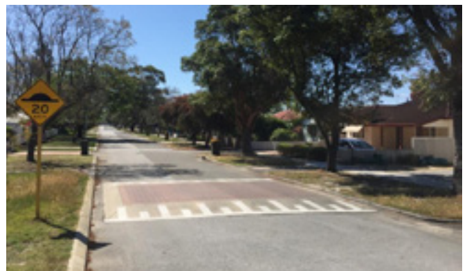
Figure 50: Raised mid-block full width flat top road hump.
