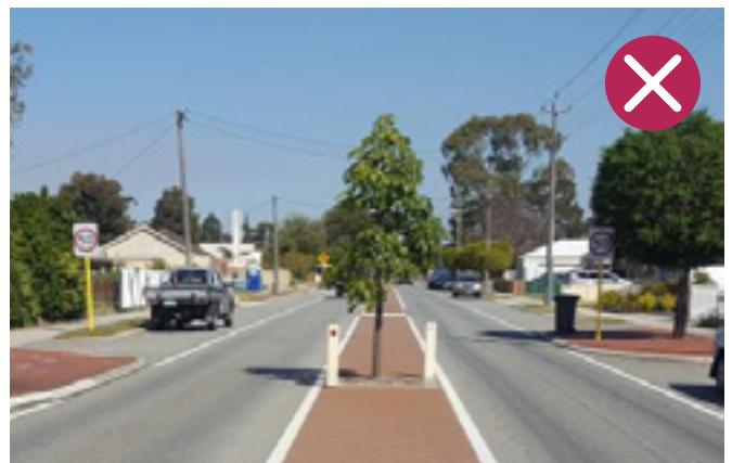
Figure 54: Flush central median with street trees.
