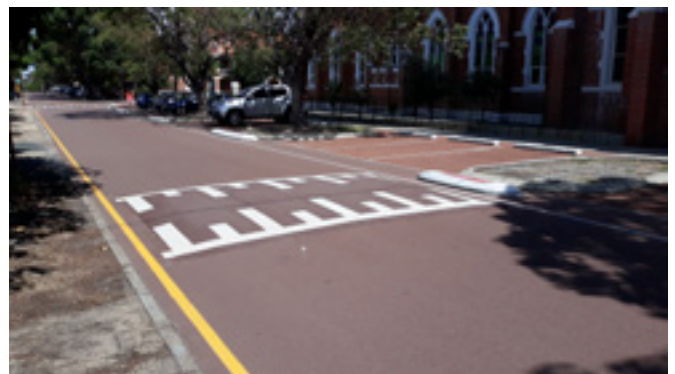
Figure 59: Kerb extension treatment.
