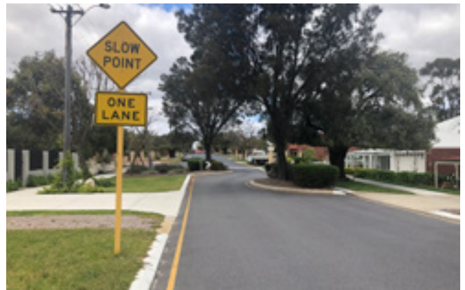
Figure 26: Single lane angled slow point.
