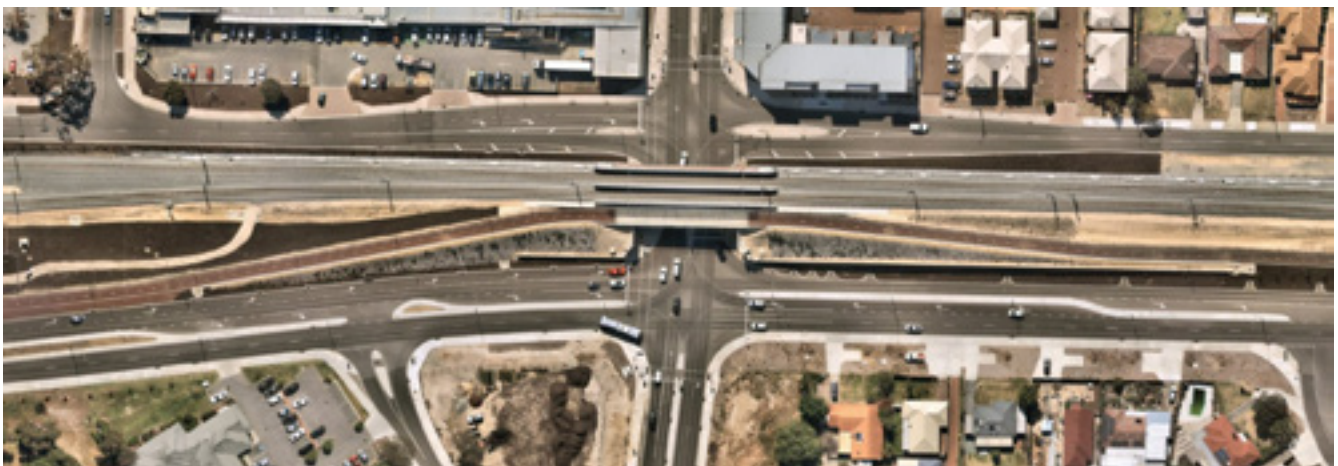
Figure 18: Shared path over Davis Road, completed as part of the Denny Avenue Level Crossing Removal project.
