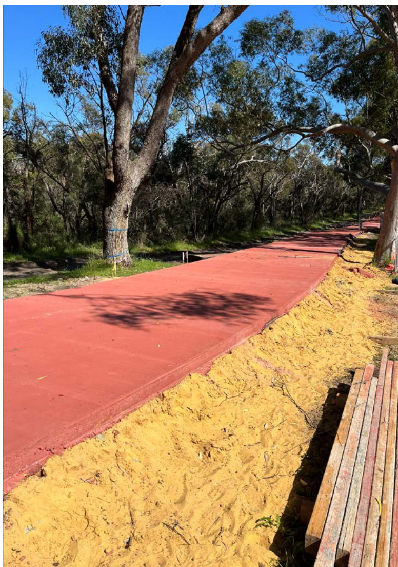
City of Perth – Construction commenced for Kings Park Road Shared Path
