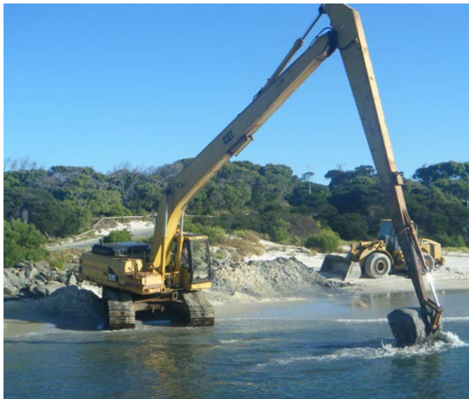
Excavation from shore – Bremer Bay 2010
