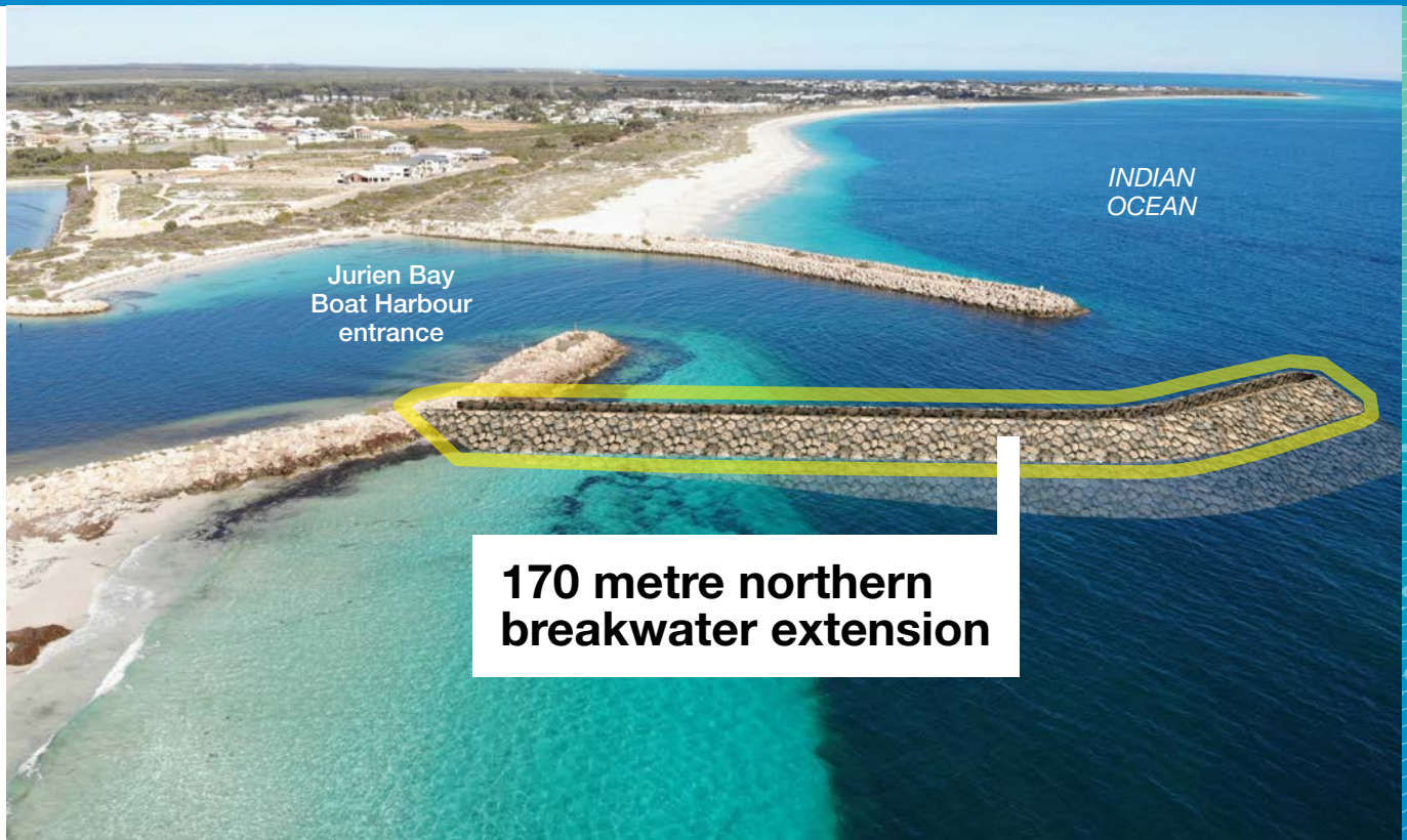
The Jurien Bay Boat Harbour northern breakwater extension
