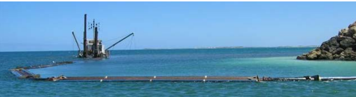
Dredging at Jurien Bay Boat Harbour
