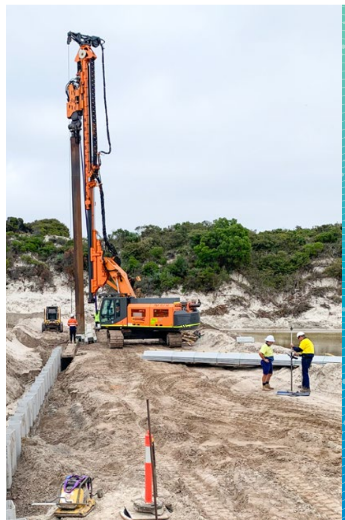
Image: Sheet piling Bandy Creek Weir reconstruction.
