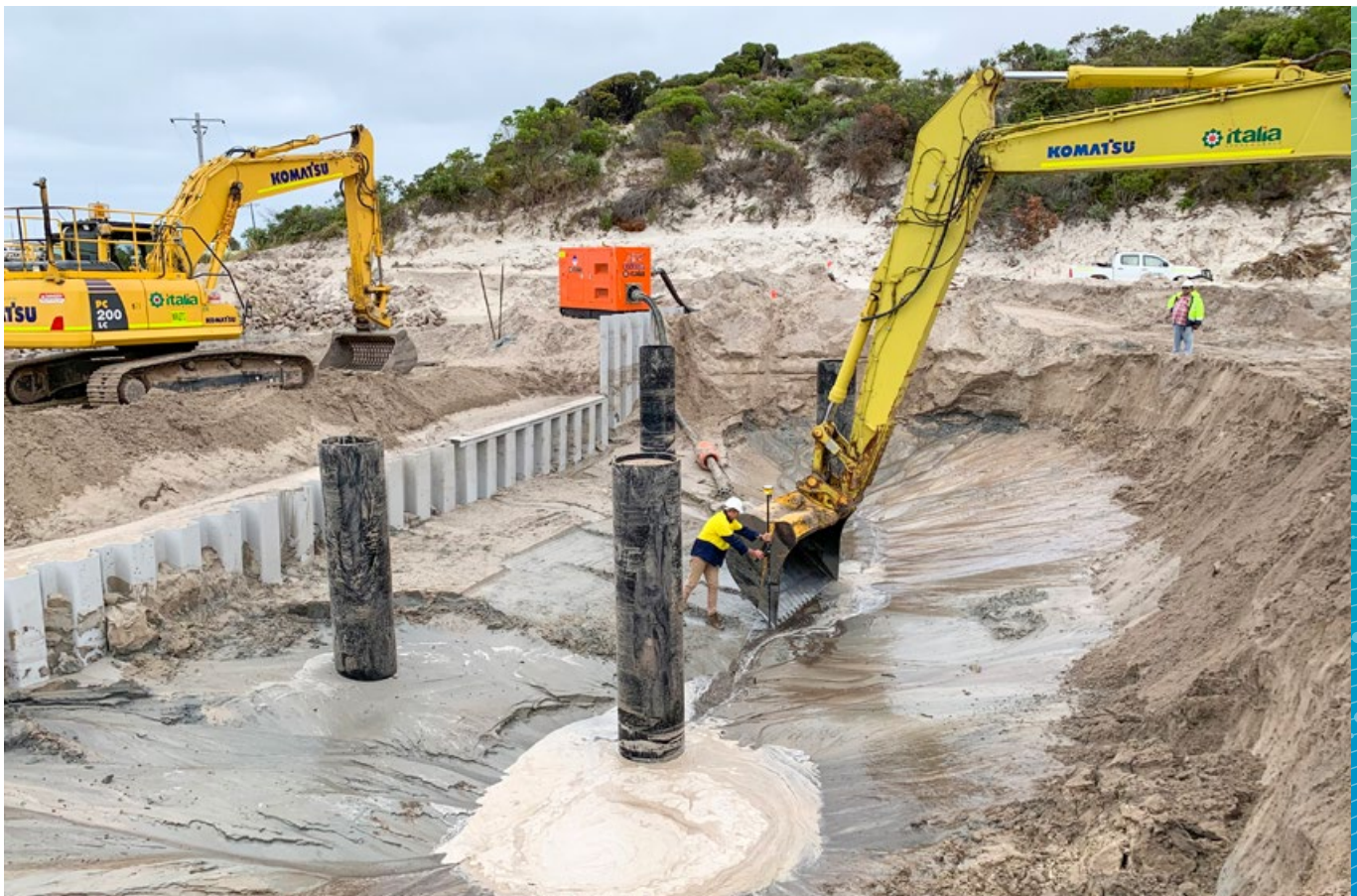
Image: Excavation works at Bandy Creek Weir reconstruction
