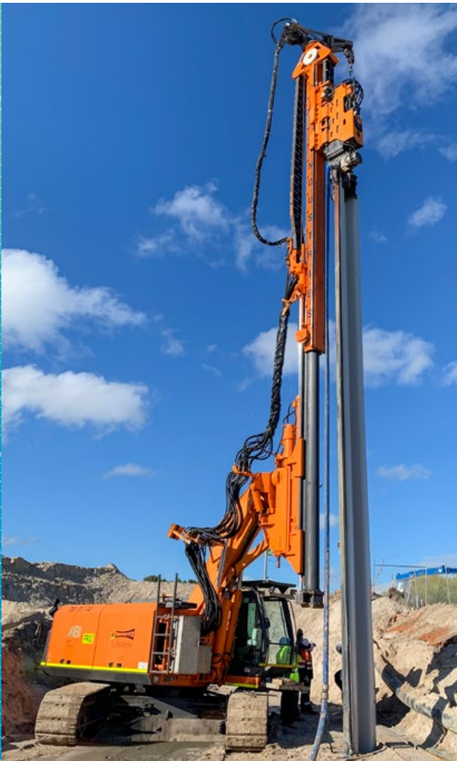
Image: Sheet piling Bandy Creek Weir reconstruction
