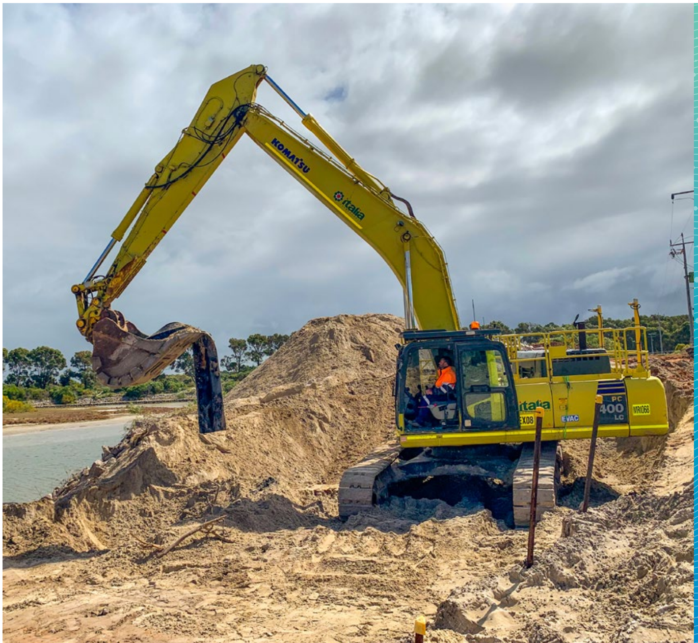
Image: Excavation works at Bandy Creek Weir reconstruction
