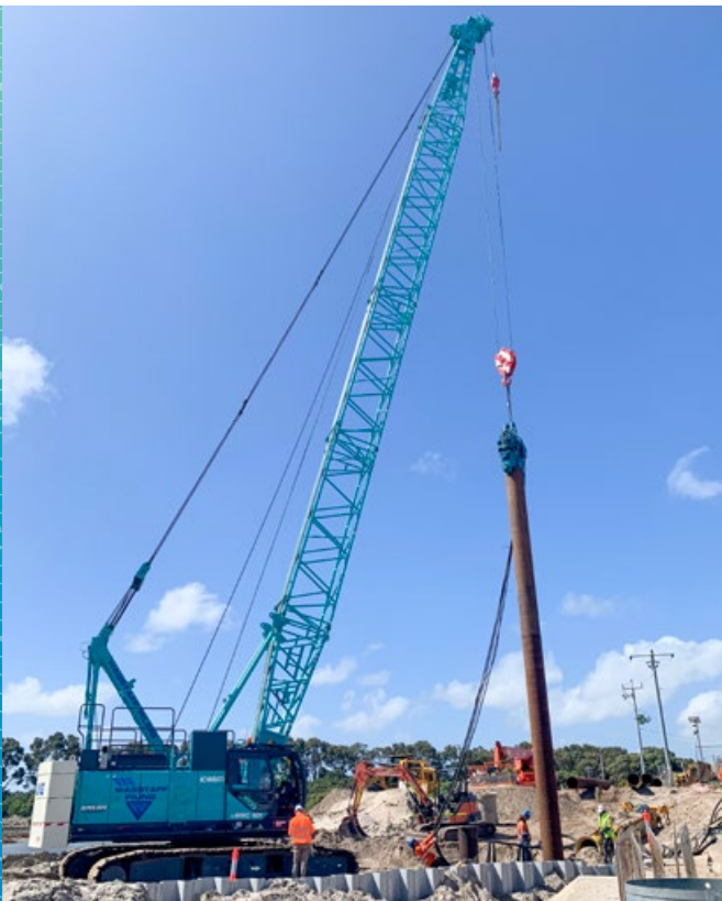
Image: Tubular piling Bandy Creek Weir reconstruction
