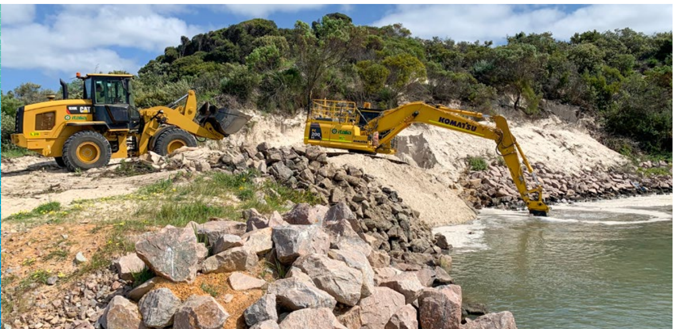
Image: Excavation works at Bandy Creek Weir reconstruction
