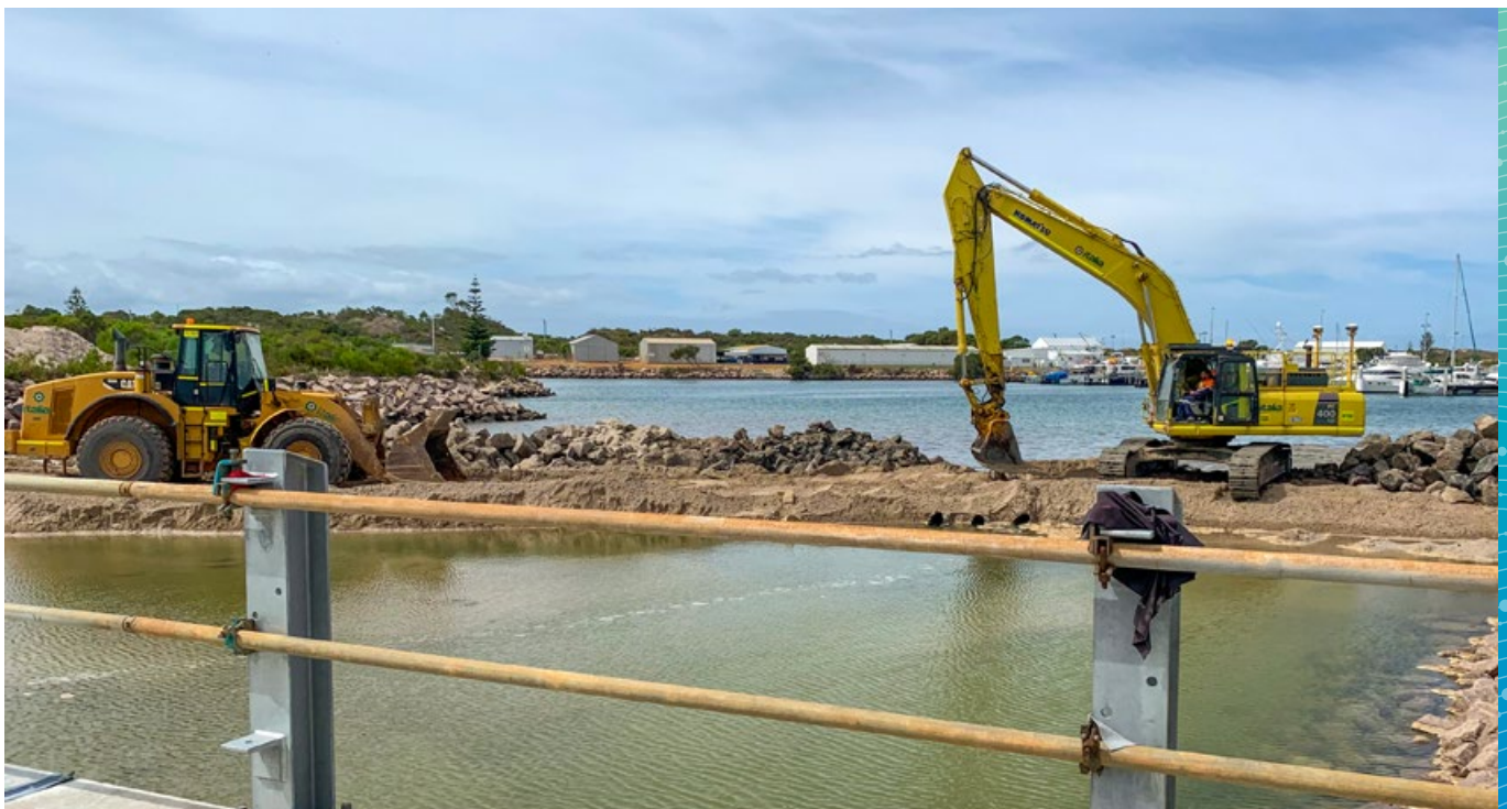
Image: Excavation works at Bandy Creek Weir reconstruction
