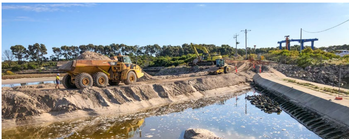
Image: Excavation works at Bandy Creek Weir reconstruction
