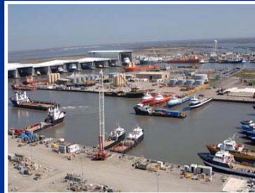
Mooring and lay down facilities
