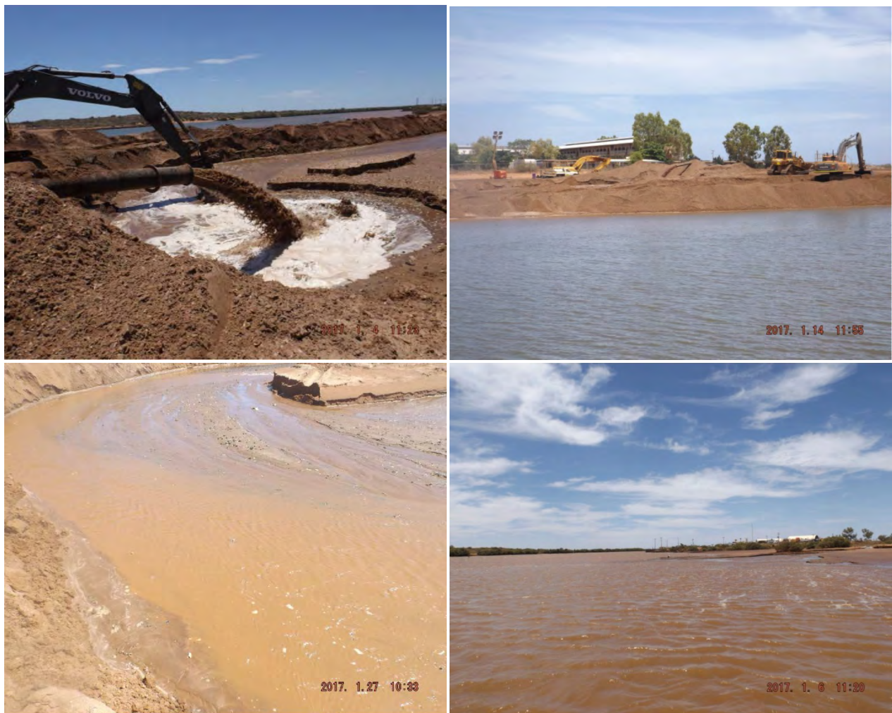
Figure 3.1 Disposal of dredged sediment to the bunded swale settlement system during the Beadon Creek 2016/17 Capital Dredging
