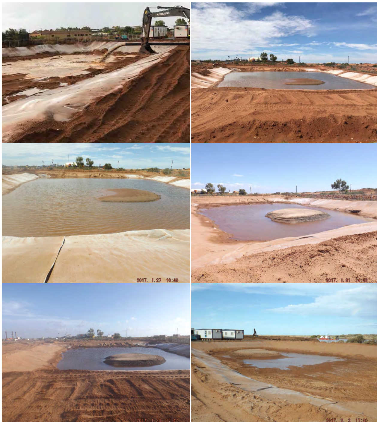
Figure 3.2 Disposal to TBT containment area (Top panel–26 January 2017) and subsequent natural dewatering during Beadon Creek 2016/17 Capital Dredging
