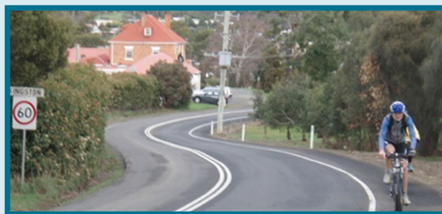
Figure 4.25 Before this project, Bonnet Hill was a narrow road with blind corners. The addition of a sealed shoulder on the uphill stretch improved safety for all road users.
