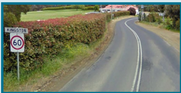
Figure 4.25 Before this project, Bonnet Hill was a narrow road with blind corners. The addition of a sealed shoulder on the uphill stretch improved safety for all road users.
