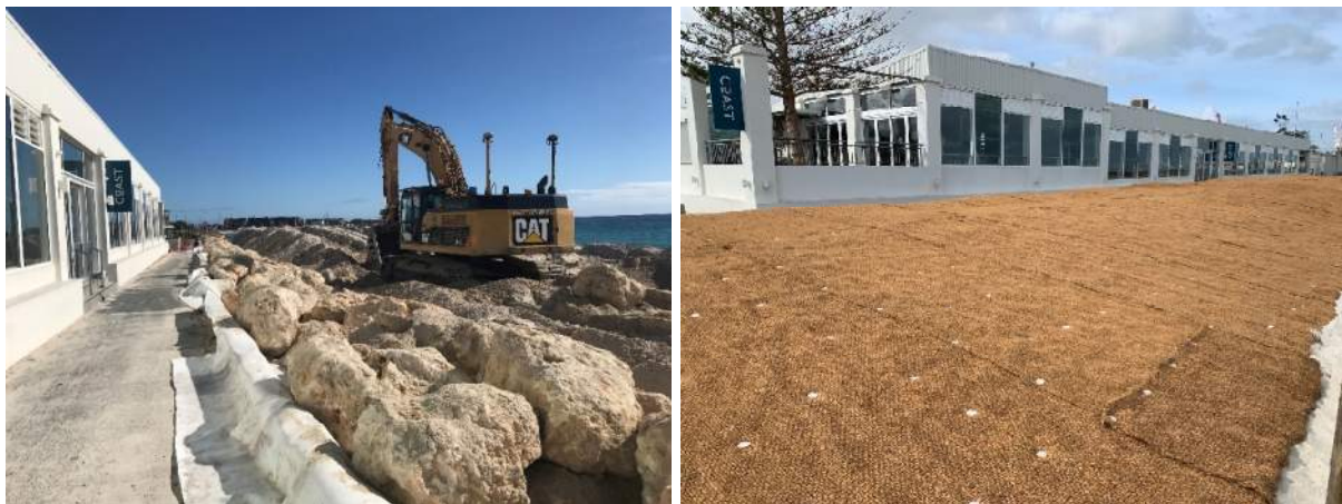
Figure 4.7 Port Beach Temporary Seawall
