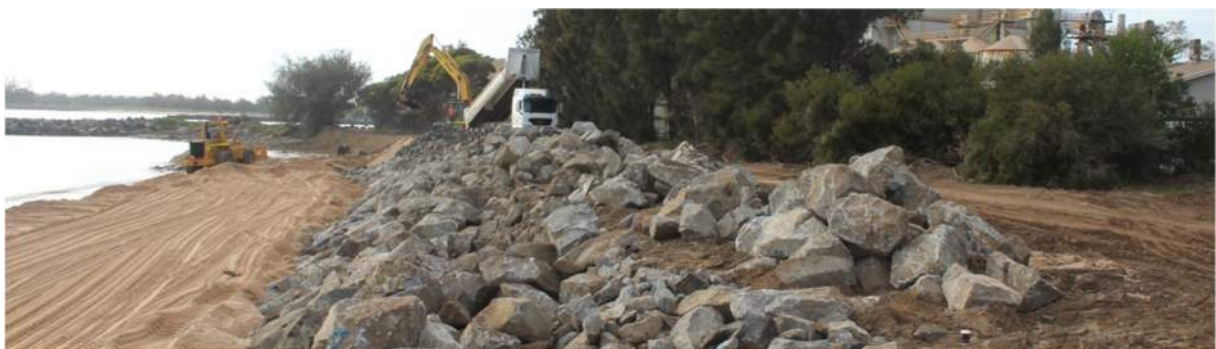
Figure 4.9 Point Busaco Revetment
