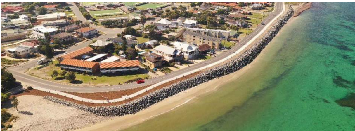
Figure 4.6 Mersey Point Seawalls (Westpeak Engineering)
