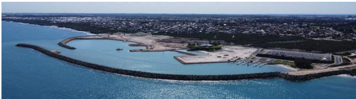
Figure 4.5 Ocean Reef Marine (ORM) Breakwater Construction
