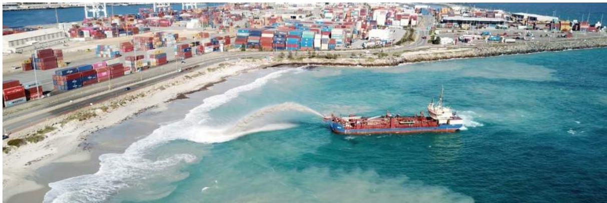
Figure 4.3 Port Beach Sand Nourishment via Dredging Works
