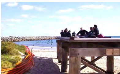
Remnant Long Jetty piles and structure
