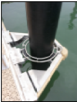
Figure 3: Typical Mooring Ring on Pile Guide (left) and Floating Mooring Ring (right)
